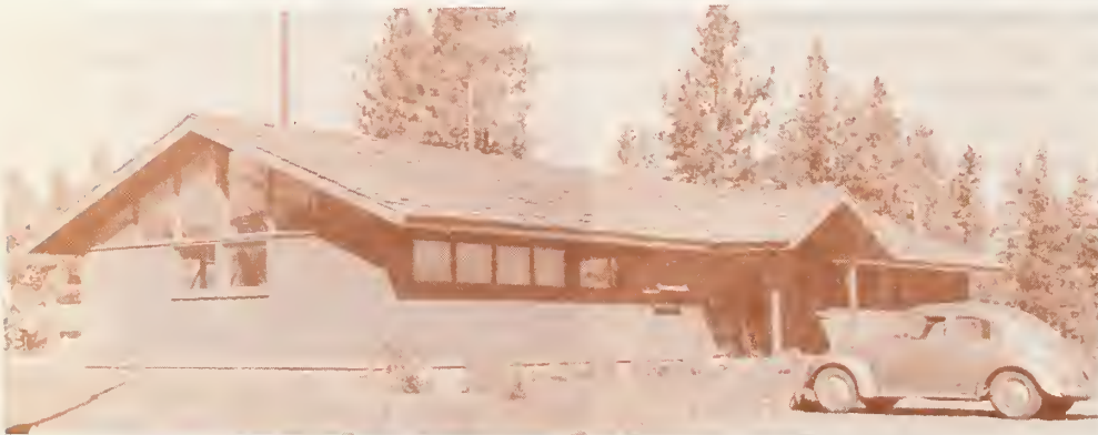
One of the new offices constructed under the expanded housing program.
