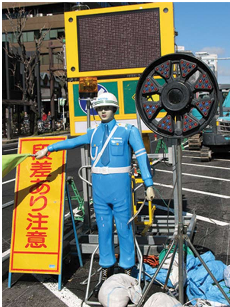
Mechanical Police at Construction Sites
