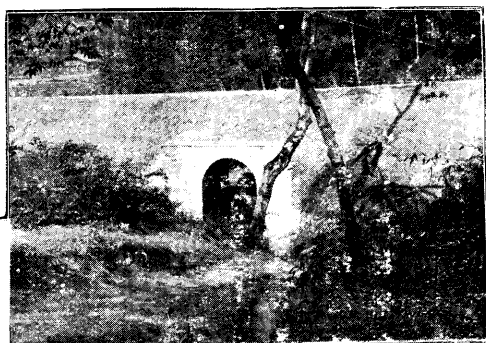
Right—One of the Culverts—Anhui Section.
