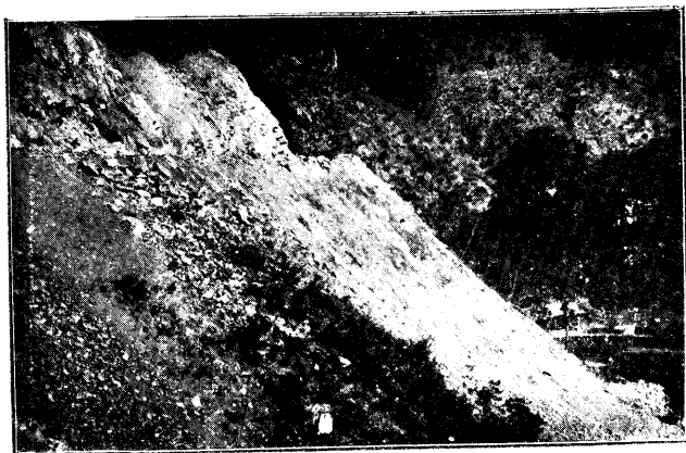
Above—Rock Excavation at Laochuling— Anhui Section.
