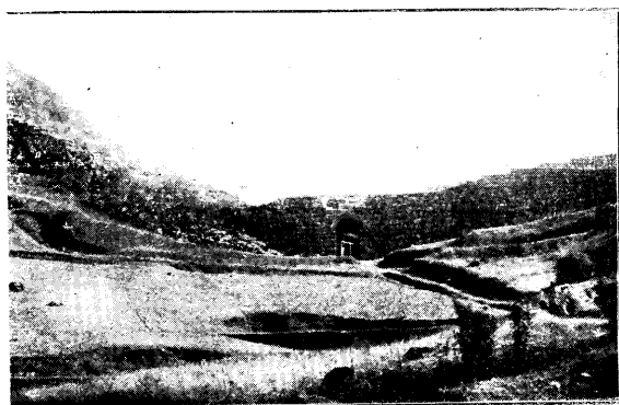
Above—Yulingkwan before Demolishing.
