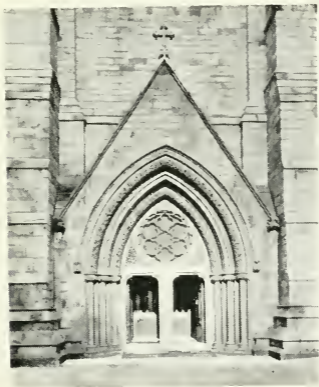
THE SOUTH PORCH.
