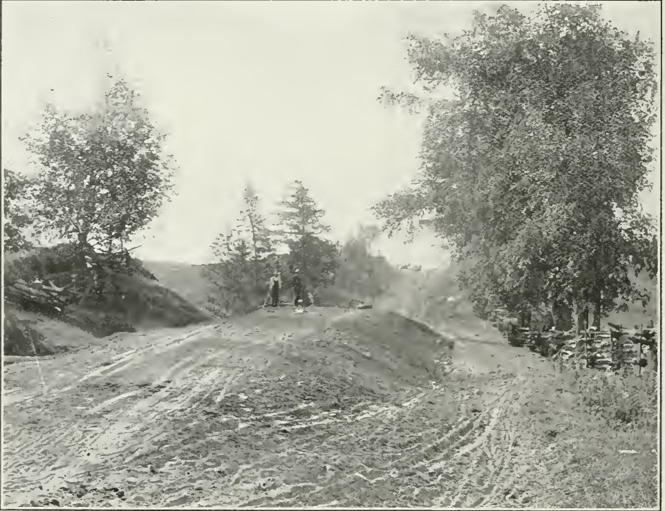
Hill Improvement in Peel County—Commencement.
