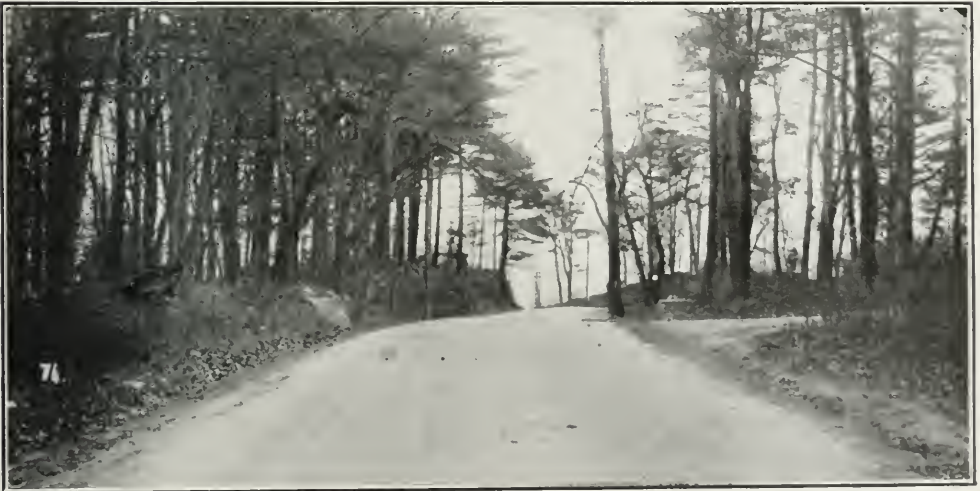
On the Massachusetts State Highway System. Treated with Asphalt Binder.
