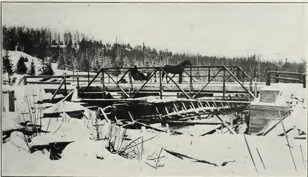
Bridge over Wissi-Wassa River, Himsworth Township.
