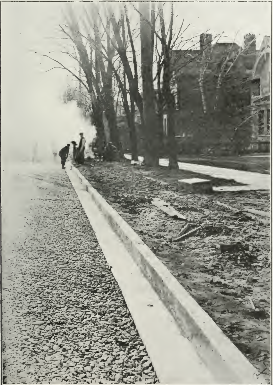
A Combined Concrete Kerb and Gutter in Ottawa.
