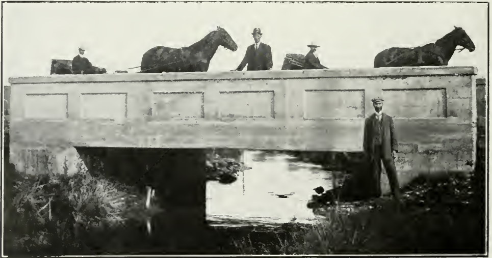
Reinforced Concrete Beam Bridge over the Credit near Orangeville. Clear Span, 22 feet; Length over all, 34 feet; Clear Width of Roadway, 20 feet; Height of Walls, 13 feet 6 inches. Walls, Floor, and Girders are Concrete, Reinforced with Steel Rods. Cost—Concrete, $448.00; Steel Reinforcing, $85.00.
