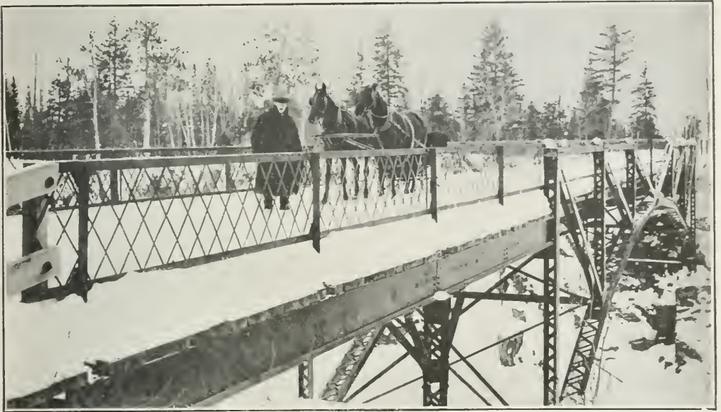
Tunnel Bridge, Mississauga River, Wells Township.
