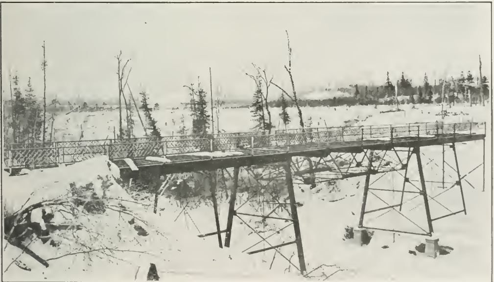
Sudbury-Soo Trunk Wagon Road over Birch Creek, near Webbwood.
