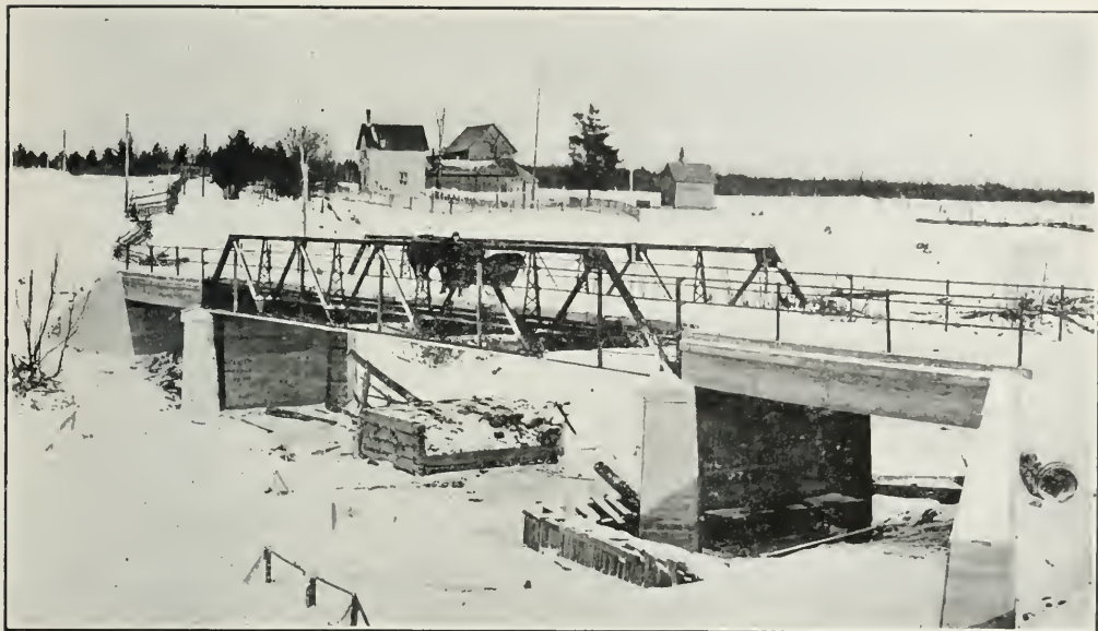
South River Bridge at Nipissing Village.
