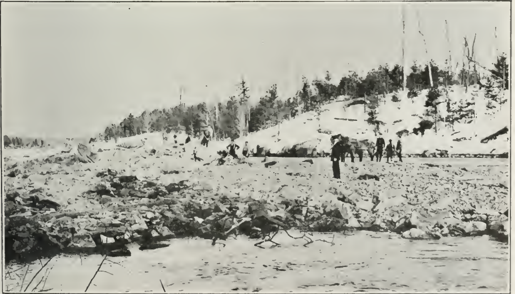
Removing Rock at Moon Chute, Muskosh River, below Bala.
