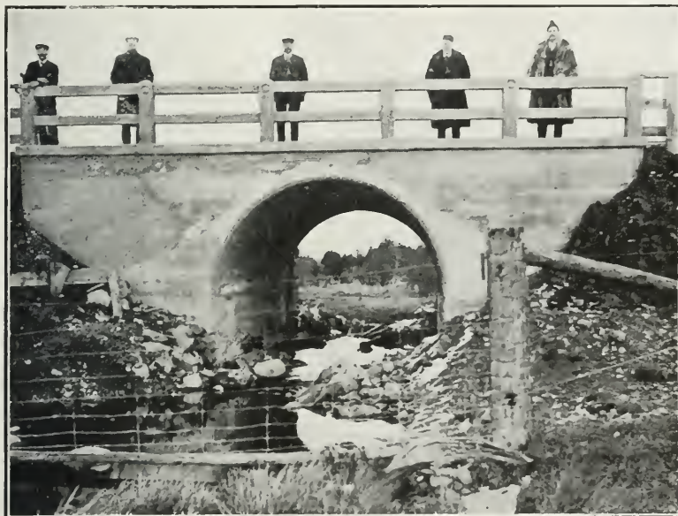
A Wellington County Bridge, near Guelph. The hand-rail is of concrete.
