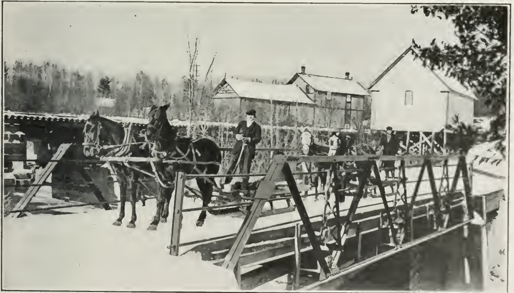
Eau Claire Bridge, over Amabel-du-Fond River.
