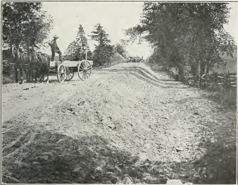
Hill Improvement in Peel County—The Completed Grade.
