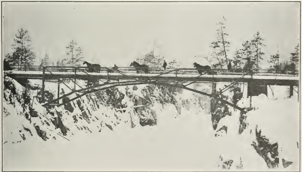
Tunnel Bridge, Mississauga River, Wells Township.
