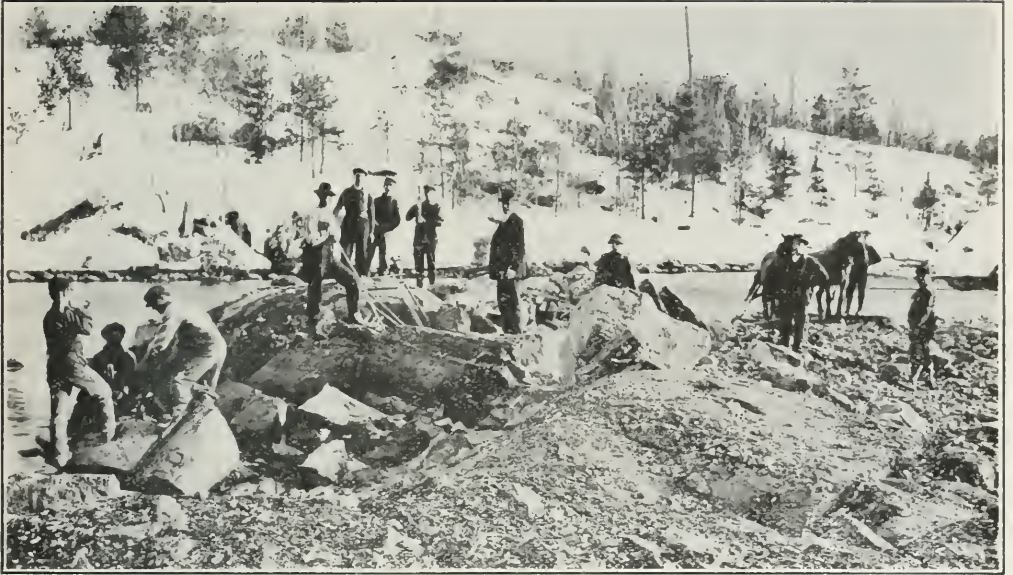
Removing Rock at Moon Chute, Muskosh River, below Bala Falls.
