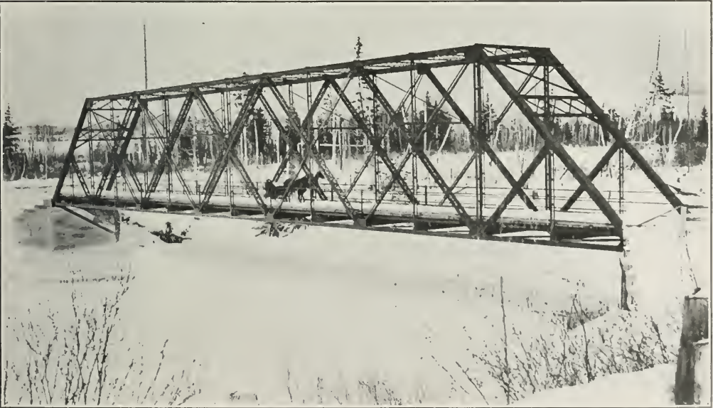
Spanish River Bridge, Nairn Township.
