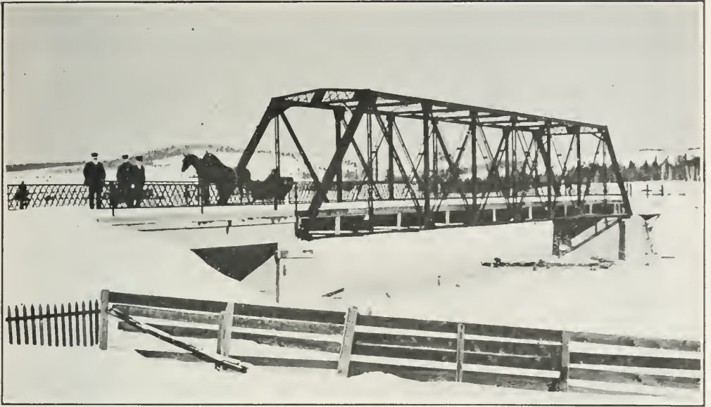
Thessalon River Bridge, at Rydal Bank.
