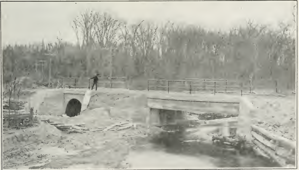
Root River Bridge, Tarentorus Township.
