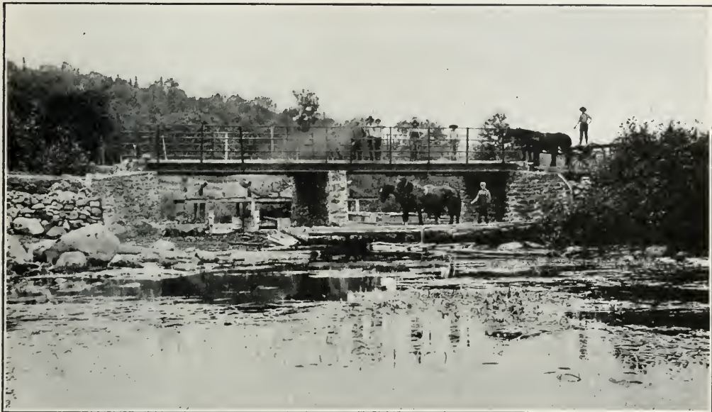
Rosseau River Bridge, Township of Cardwell.
