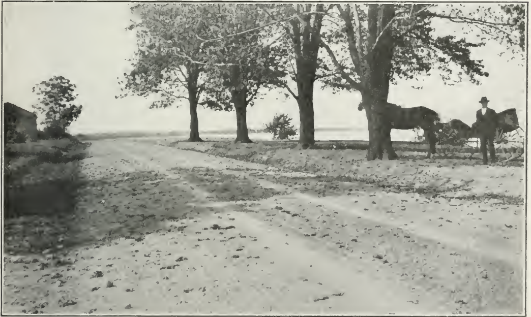
The Niagara Boulevard. A Completed Section of the Roadway.
