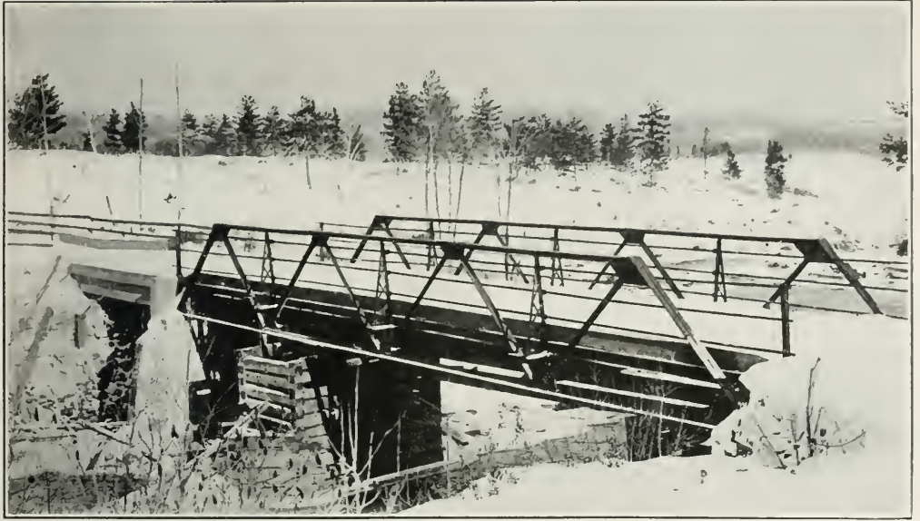
Eau Claire Bridge, over Amabel-du-Fond River.
