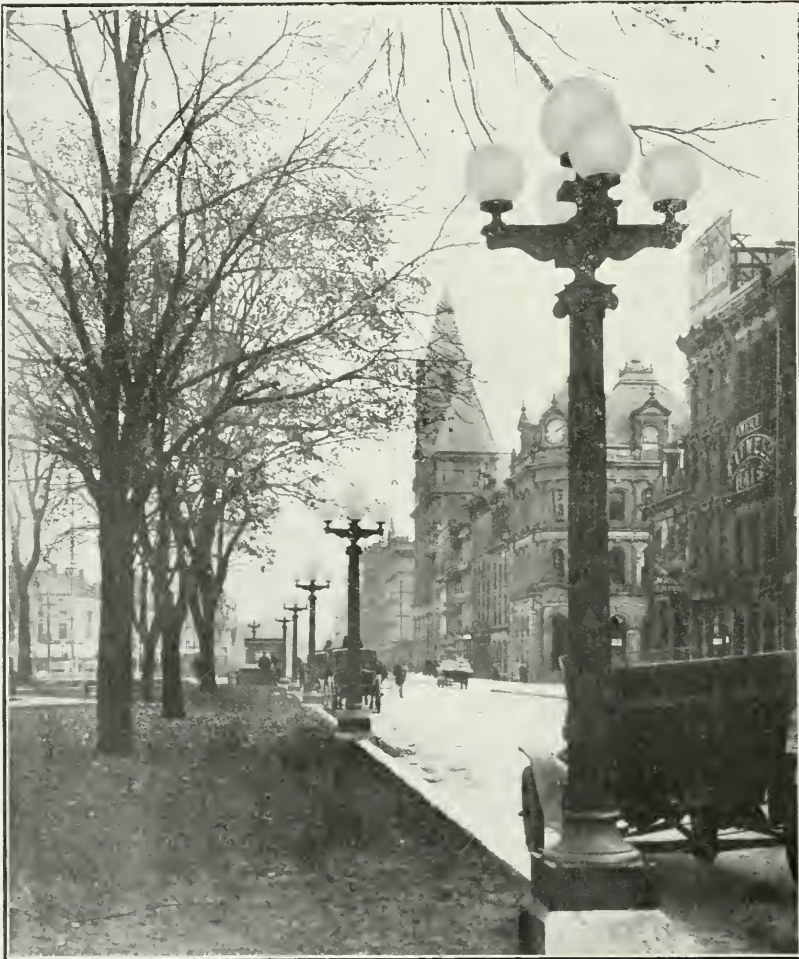
Ornamental Electric Light Posts.
