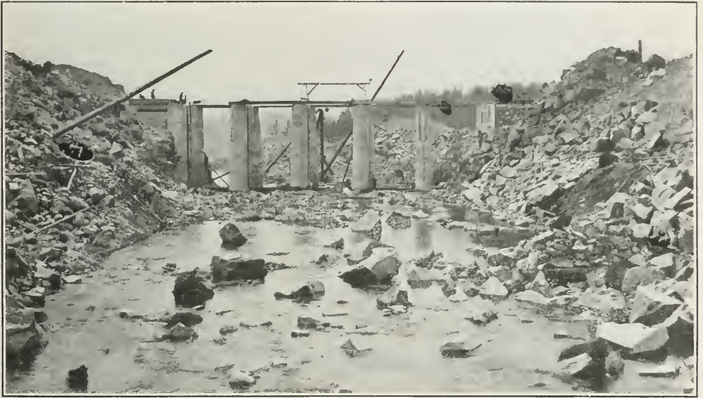
Regulating Dam at Outlet of Dog Lake, Thunder Bay District.
