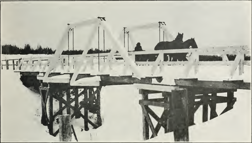
Bridge over North Branch, Veuve River, near Markstay.
