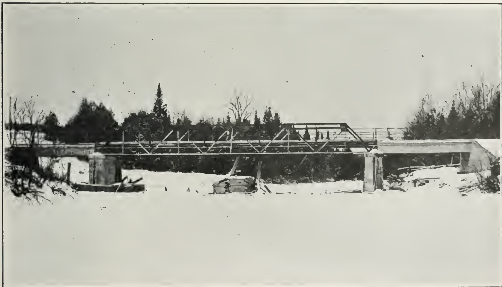
South River Bridge at Nipissing Village.
