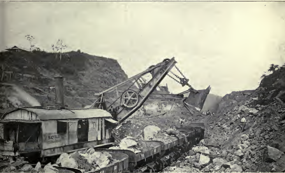
STEAM SHOVEL IN THE CULEBRA CUT.
