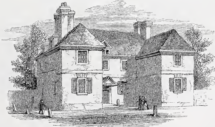
SLATE-ROOF HOUSE PHILADELPHIA.
