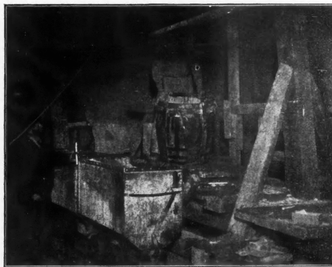
WINZE 50 FT. DEEP, NO. 3 TUNNEL LEVEL, REPUBLIC MINE, WASHINGTON.
