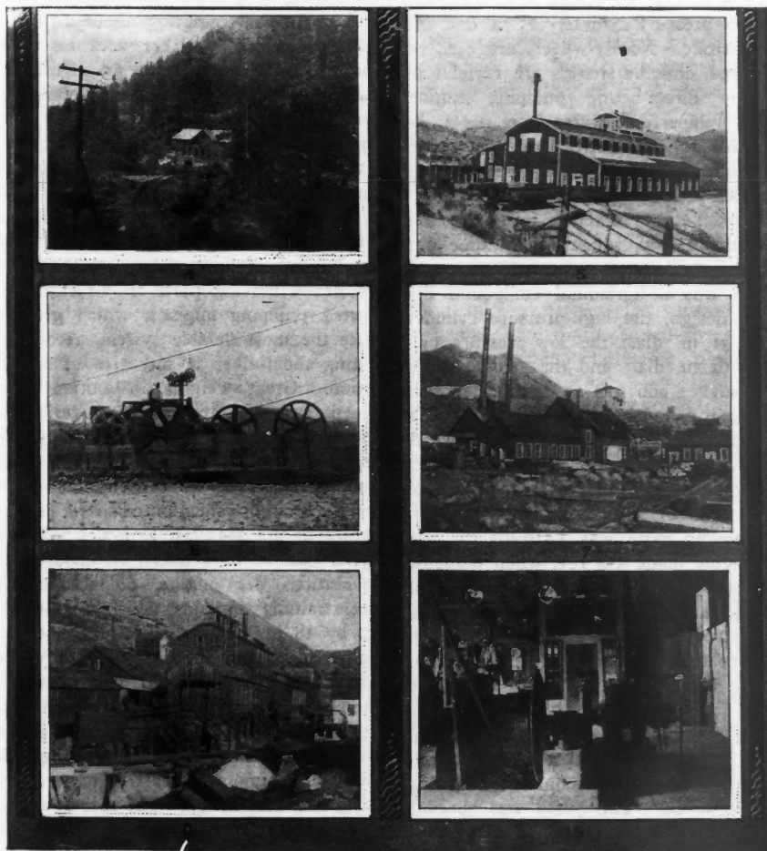
PUMPING STATIONS ON THE COMSTOCK.
