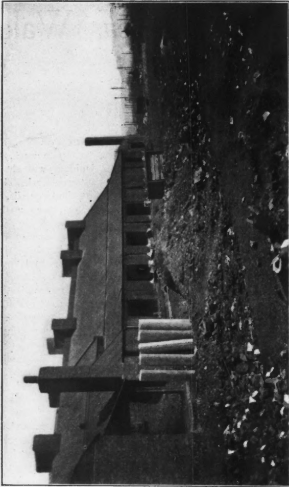
KILNS FOR HEATING. NEW RETORTS ARE SHOWN ON THE LEFT
