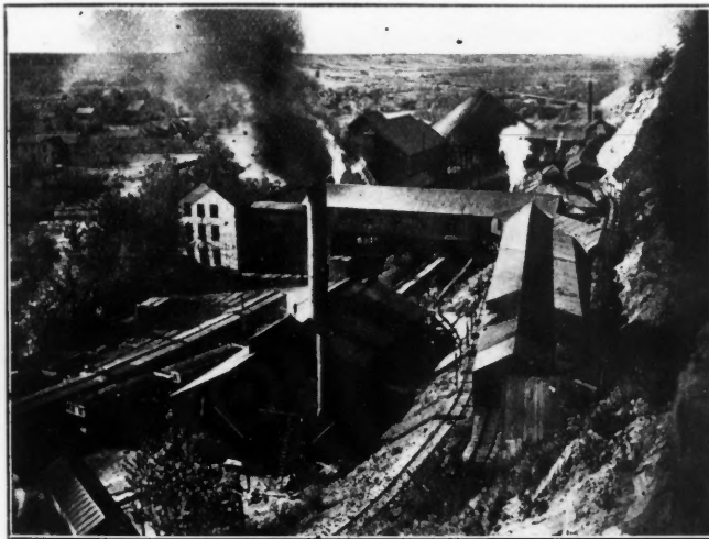
FIG. 1. NORTHERN PACIFIC PLANT AT RED LODGE, MONTANA
