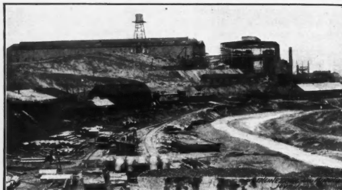
CHAMBER AND TOWER BUILDINGS DURING CONSTRUCTION
