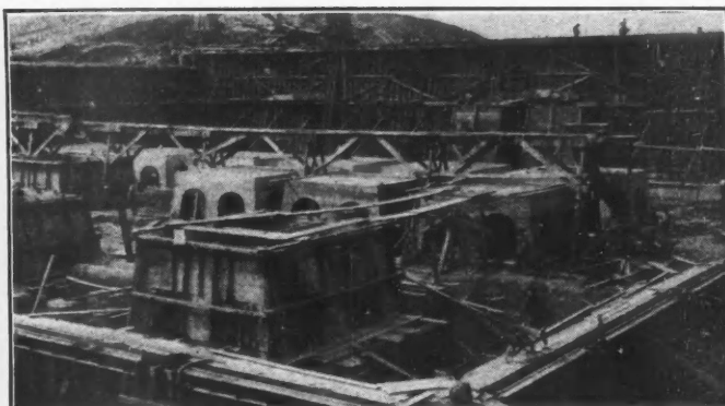
PLACING OF CONCRETE FOUNDATIONS
