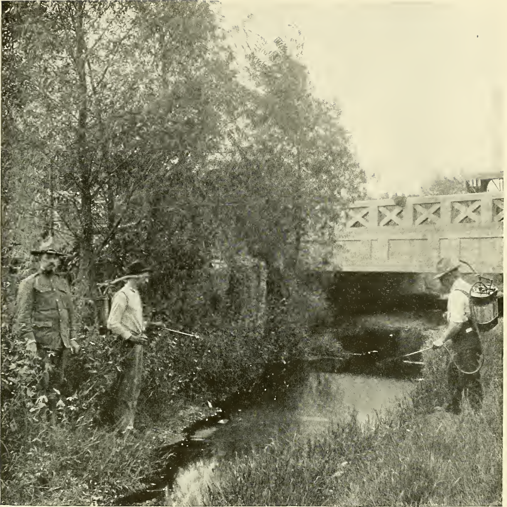
VIEW SHOWING OILING OPERATIONS FOR THE CONTROL OF MOSQUITO BREEDING
