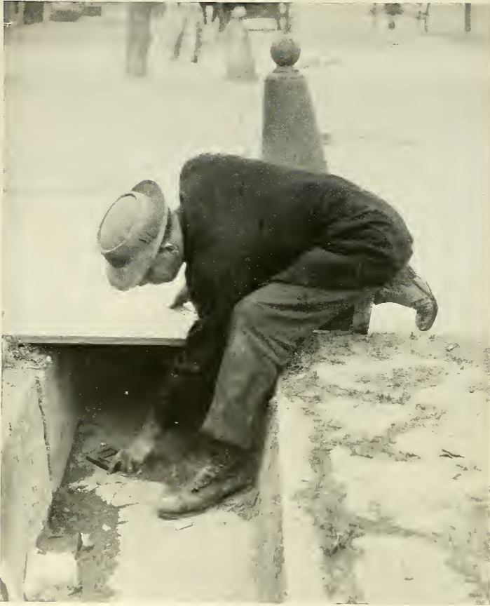
Photograph from U. S. Public Health Service SNAP-TRAPS IN SURFACE SEWERS
