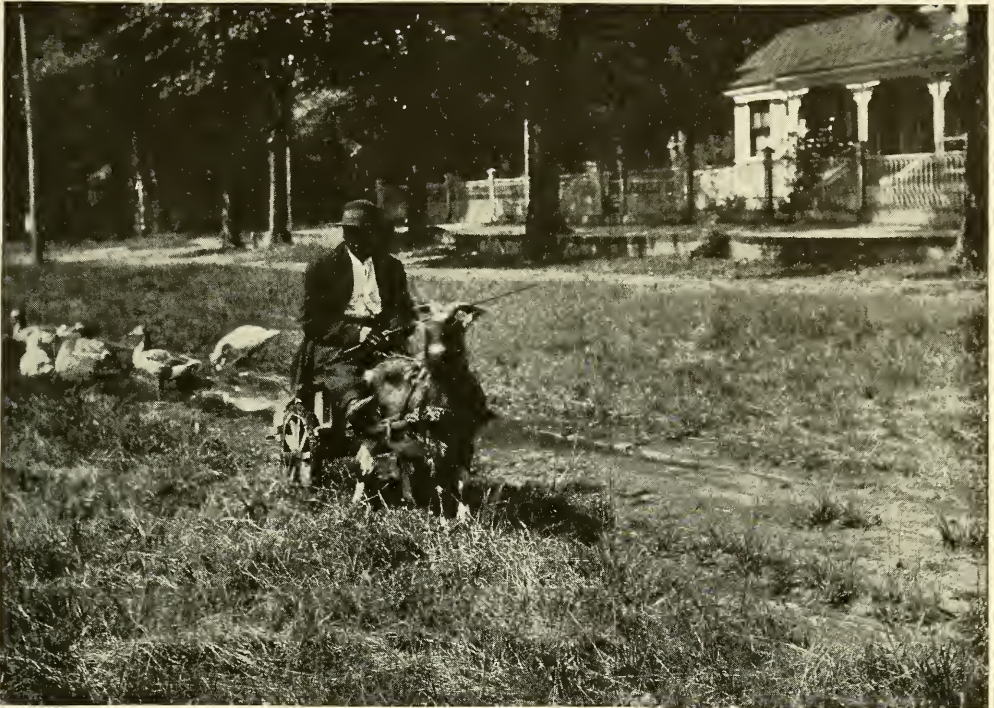
Photograph from Office of Public Roads
