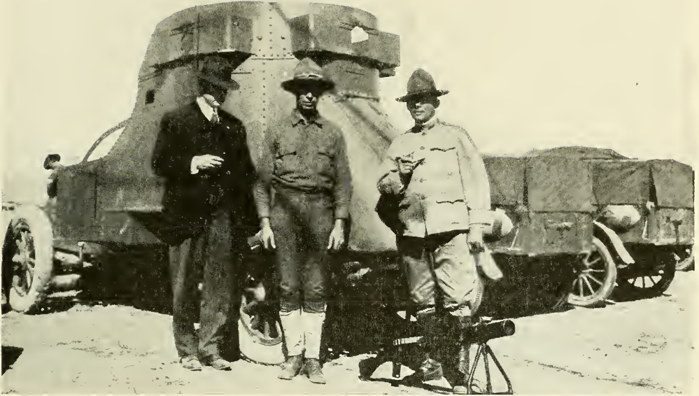
Photograph from Office of Public Roads
