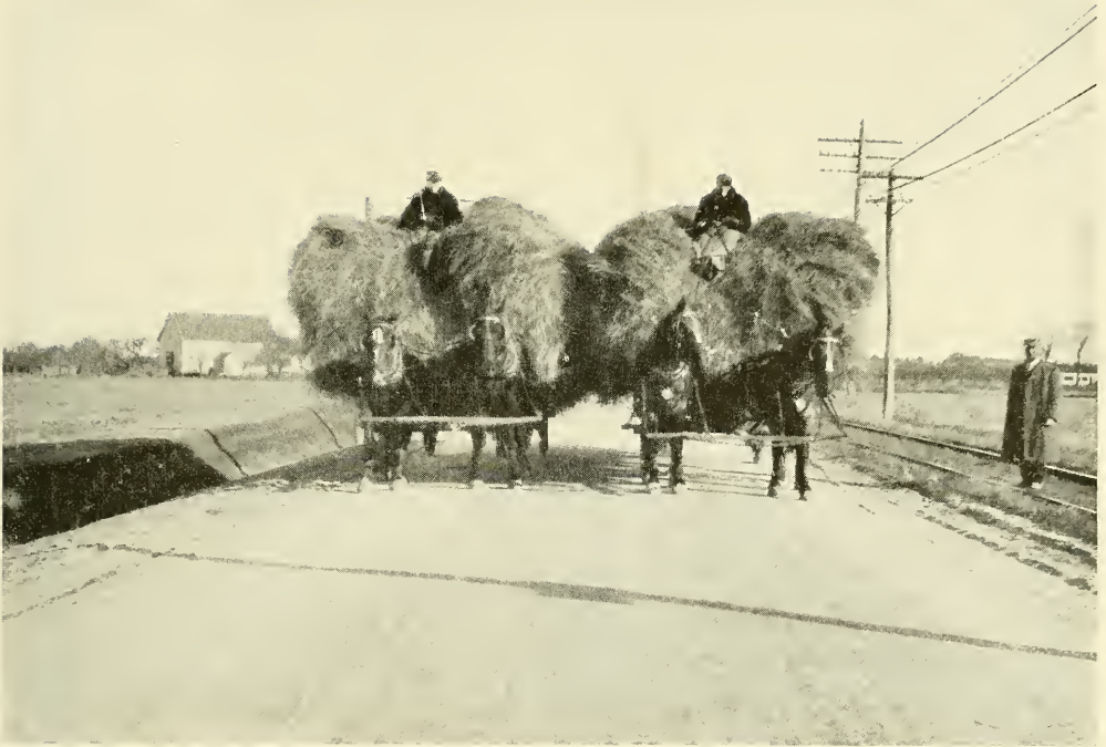
Photograph from Office of Public Roads
