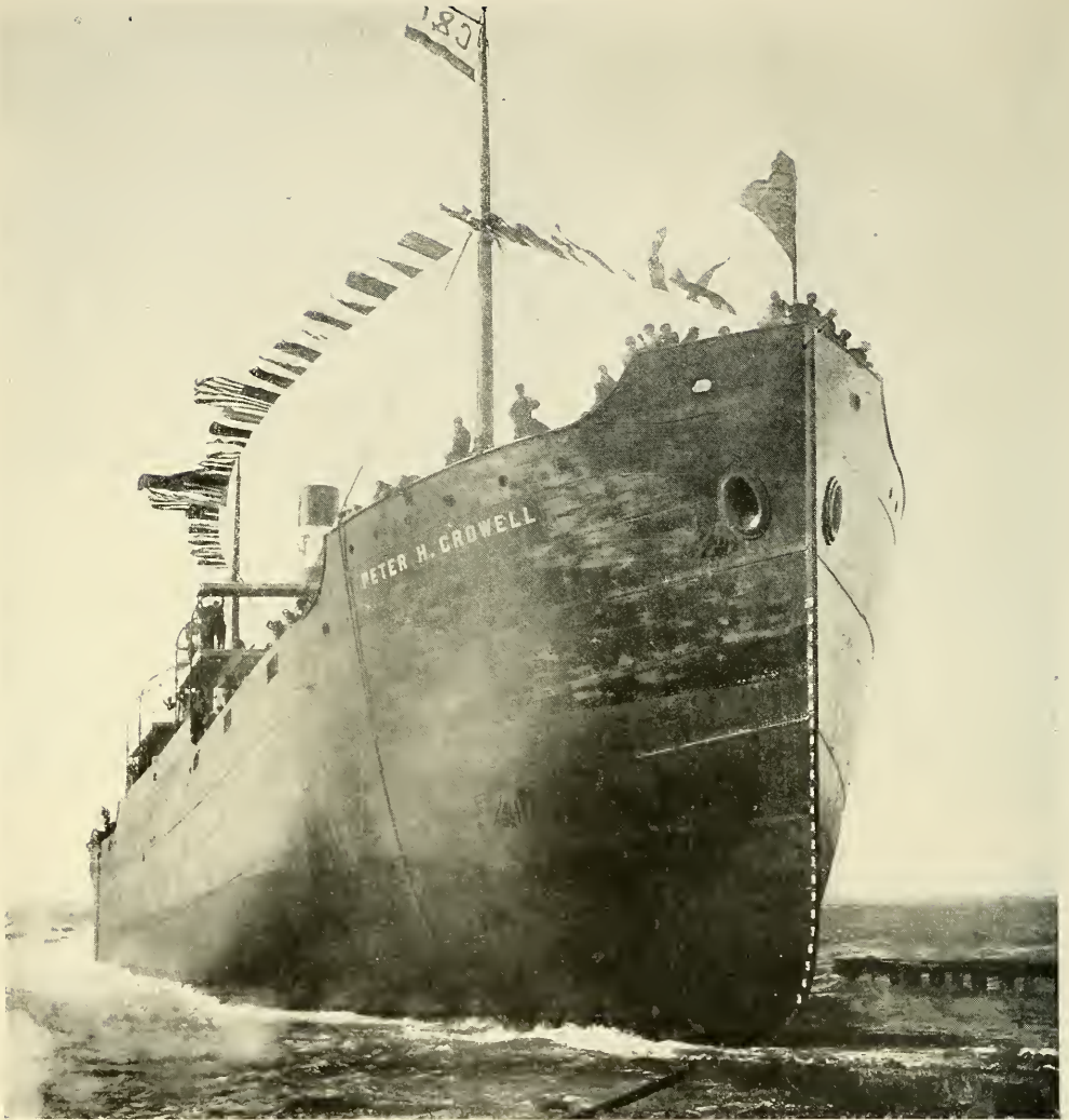
LAUNCHING A STEEL MERCHANTMAN AT NEWPORT NEWS, VIRGINIA
