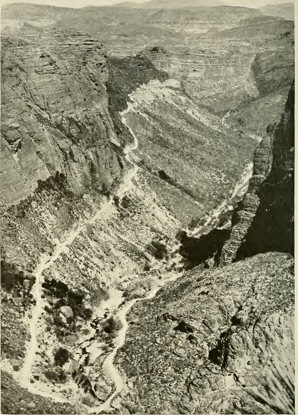
THE EAST, WEST, NORTH, AND SOUTH BECOME ONE WHEN ROADS LINK THEM A highway in one of our Southwestern States which has a grade falling 1,000 feet in one and a quarter miles
