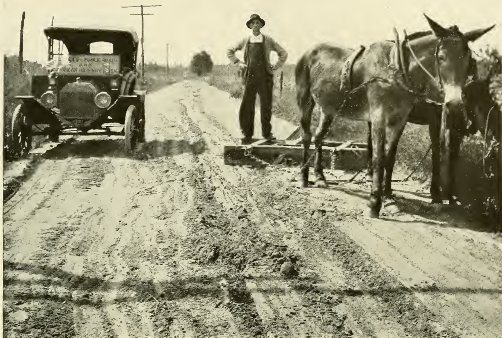
USING A DRAG IN THE IMPROVEMENT OF A ROAD IN NORTH CAROLINA
