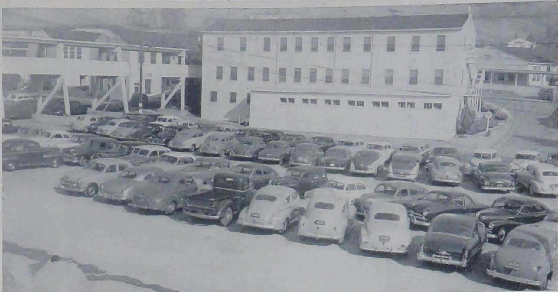
Only slightly more than two months ago, the parking area shown above was a deep and broad gully through which meandered a small stream. Now it is a large, smooth area which does much to alleviate the shortage of parking spaces on the Oak Knoll compound. Buried deep below the automobiles is a six-foot conduit through which the small stream now runs. And the dirt used to fill the gulch also created new parking areas at various spots around the compound where hills were cut away and leveled.
