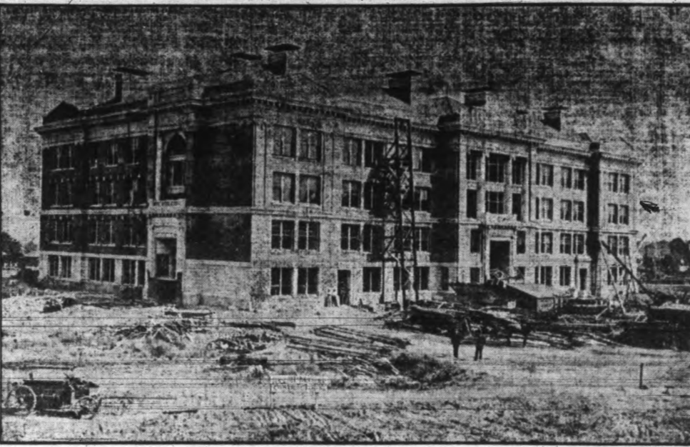
PALATIAL NEW HIGH SCHOOL WHICH WILL SHORTLY OPEN DOORS
