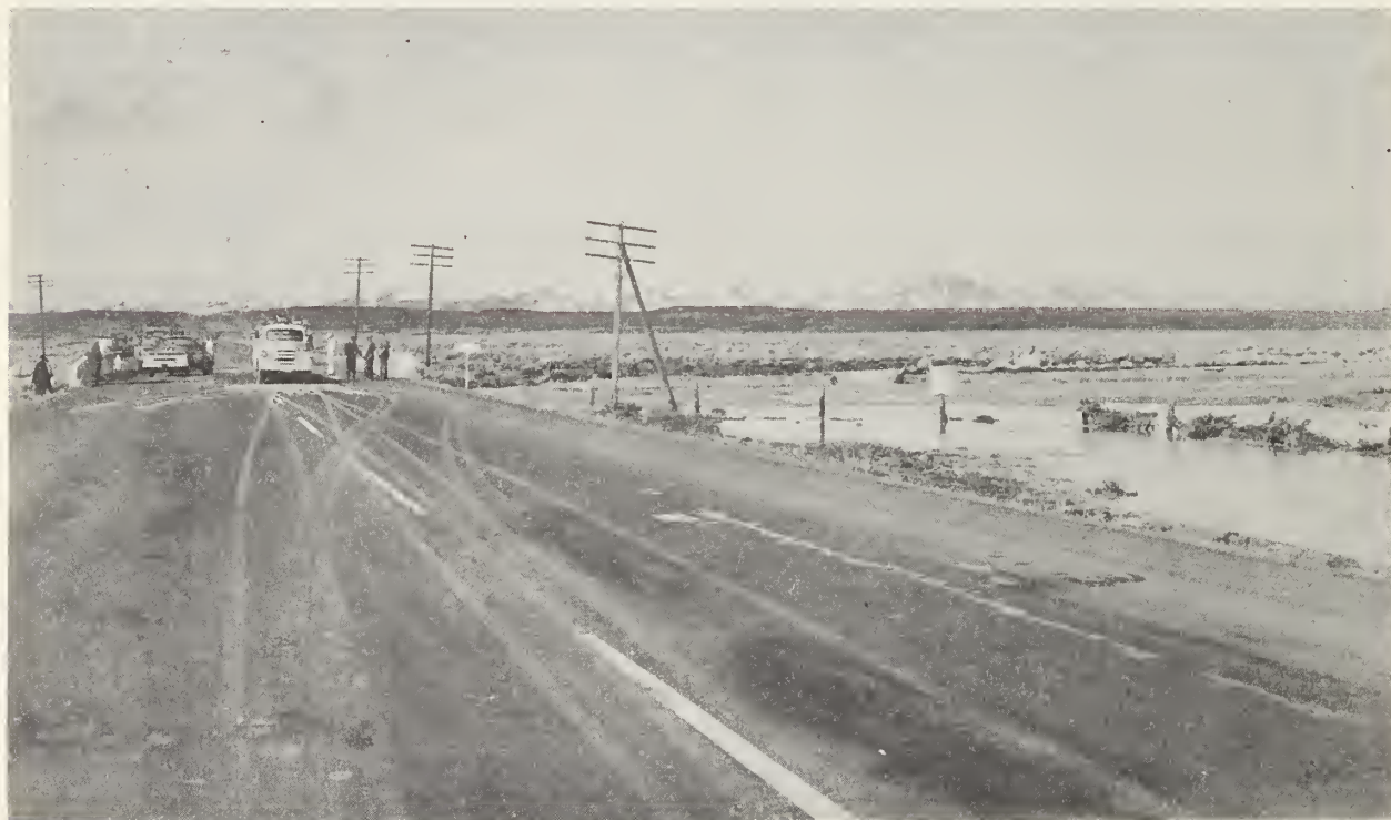
Photograph 5. - Damage to North Fork Bridge, U. S. Highway 40, February 13, 1962. Looking west.
