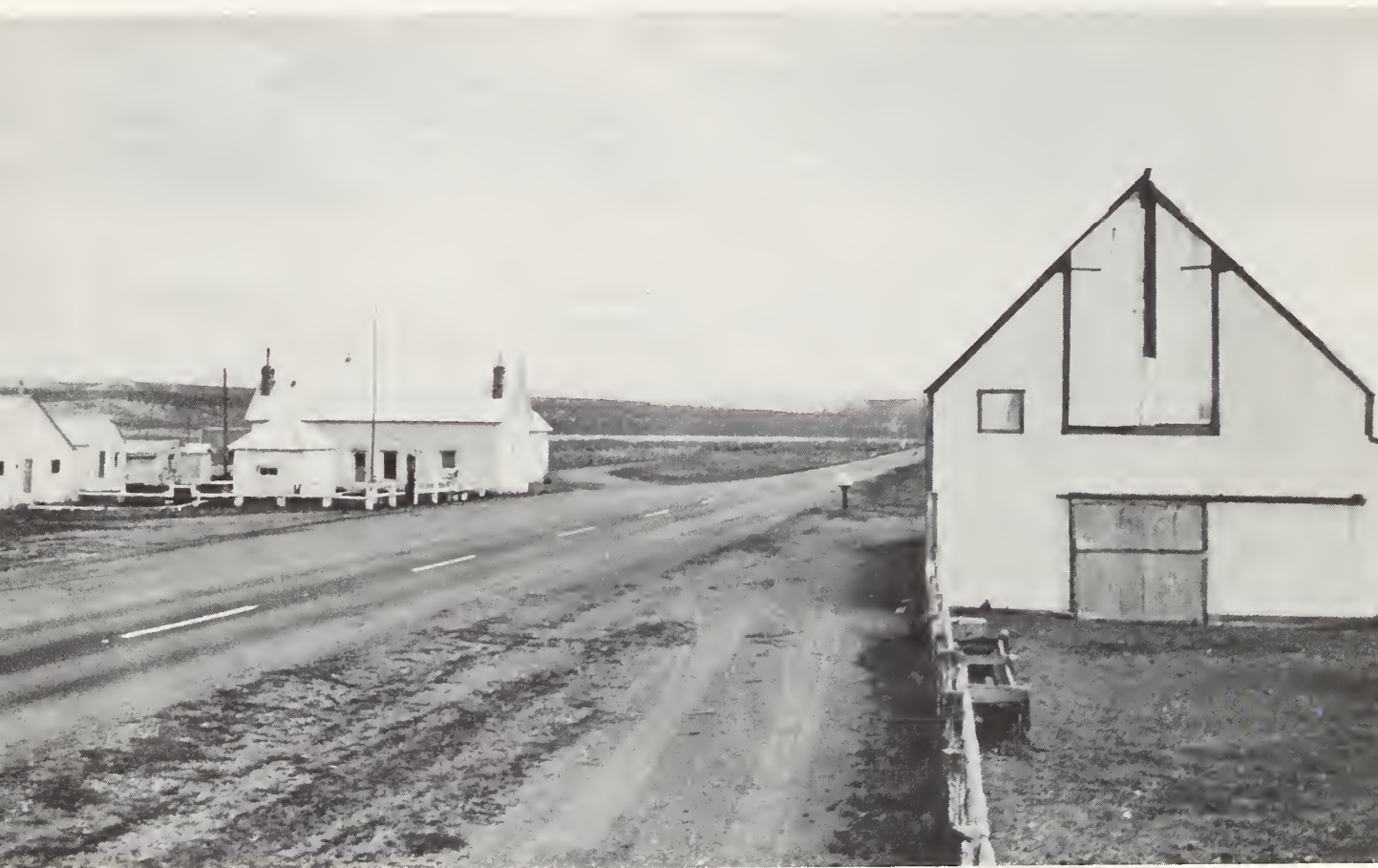
Photograph 1. - Dinner Station Ranch headquarters, Nevada Highway 11 between Elko and Mountain City, looking north. The large stone building on the left was the general store and dining room during the staging days between Elko, Mountain City and Tuscarora. The large building on the right was the barn for stage horses, changed here on all runs. The old Tuscarora stage road may be seen leaving the highway to the right of the dining room.
