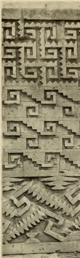
Fig. 54. Detail of Wall Construction at Mitla, showing the separately Carved Stones.
