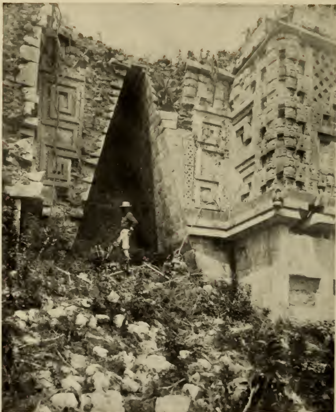
Plate XVII. A Sealed Portal Vault in the House of the Governor at Uxmal, a Building of the Second Empire, probably Thirteenth Century. The vincer character of the cut stone comes out clearly. Peabody Museum photograph.
