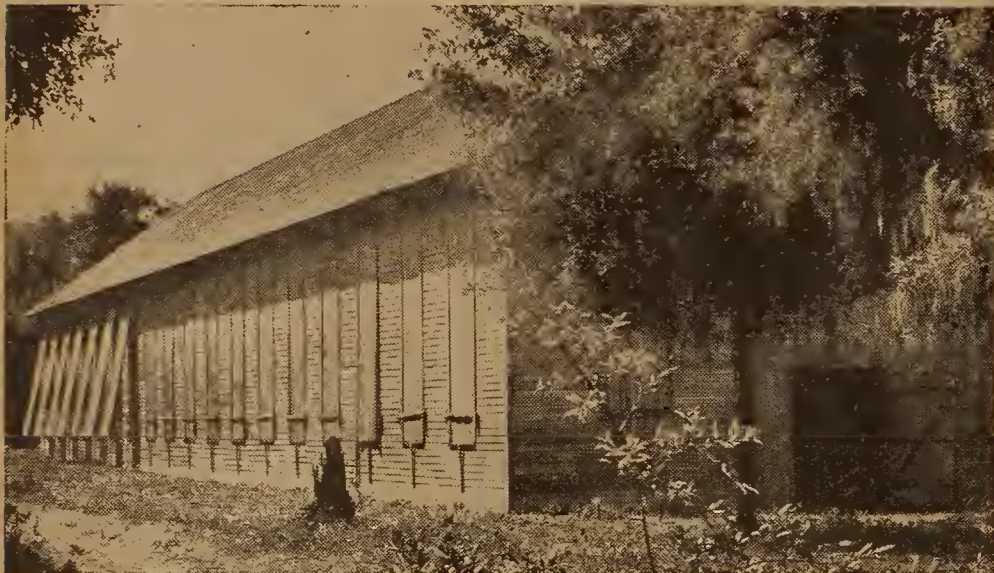
As ventilation plays a big part in curing, the barns have many windows
