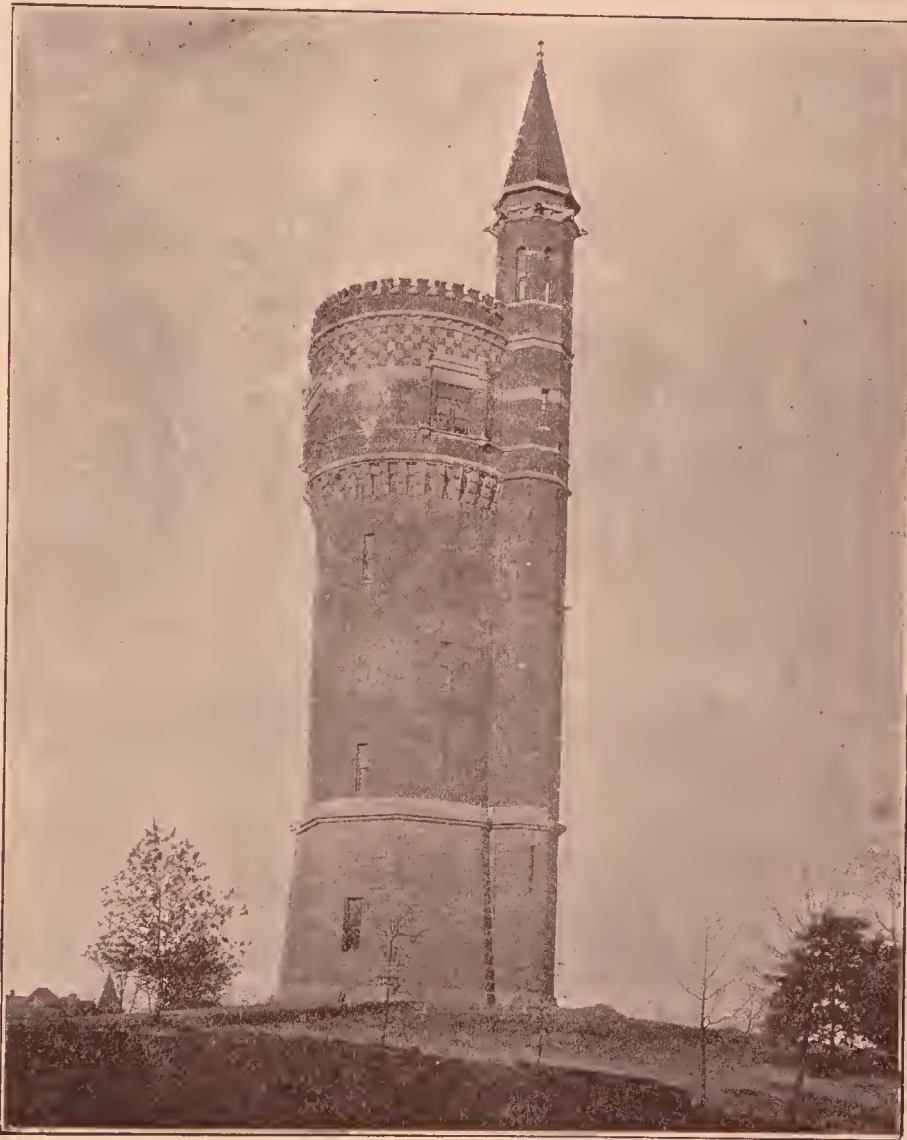
EDEN PARK WATER TOWER.
