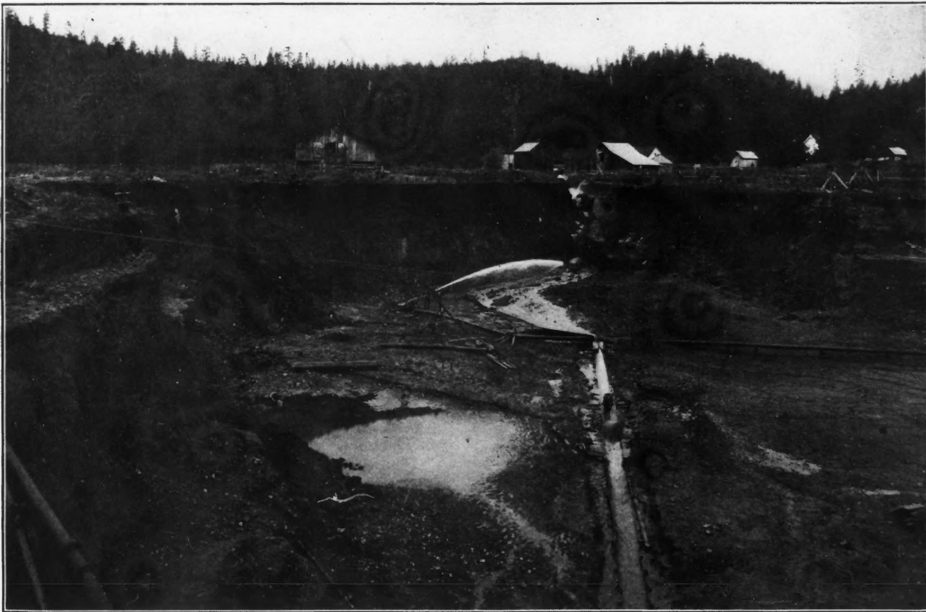
PIPING IN THE PIT OF THE LOGAN MINE, WALDO, ORE.
