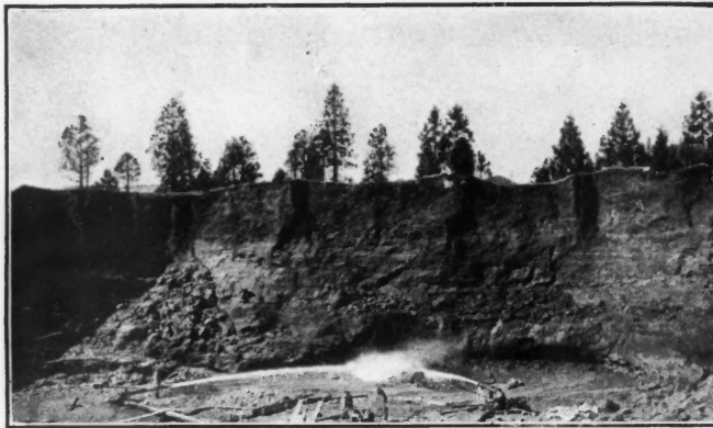
Piping in the pit of the Deep Gravel Mine at Waldo. See view of sluice and elevator below
