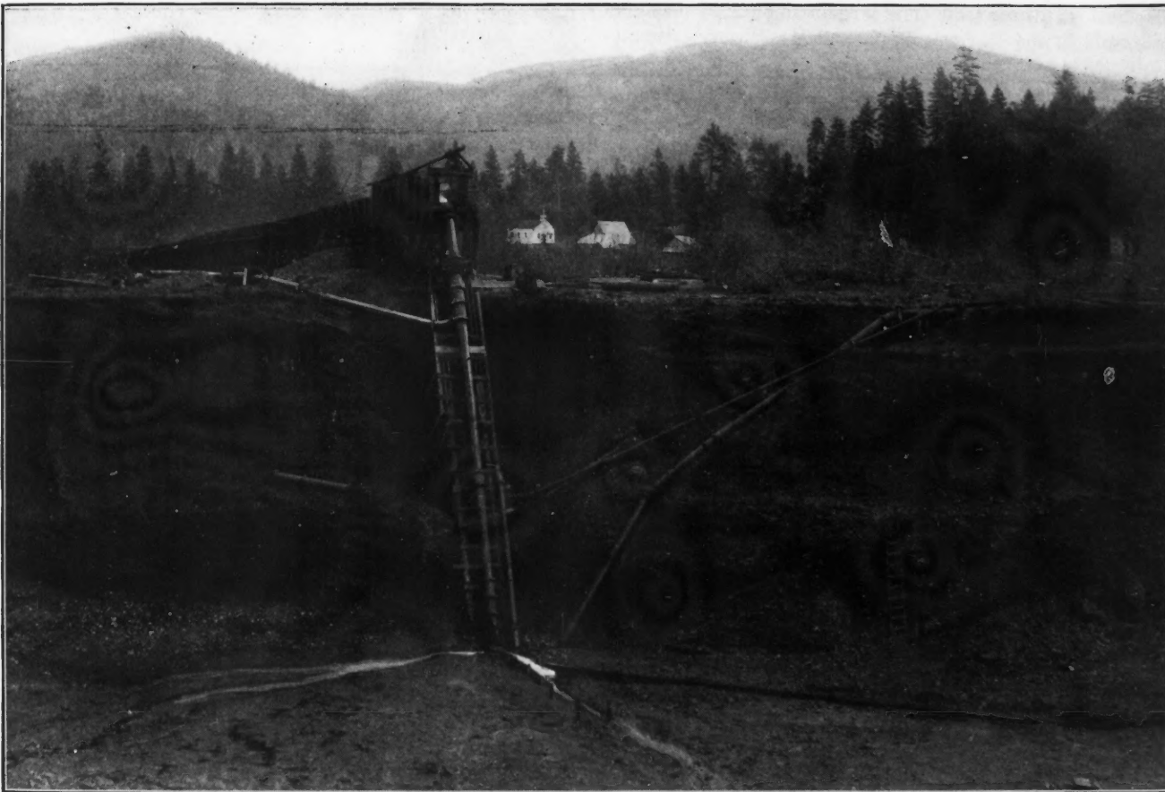
RAISING GRAVEL TO THE FLUME WITH HYDRAULIC ELEVATOR, LOGAN MINE, WALDO, ORE.
