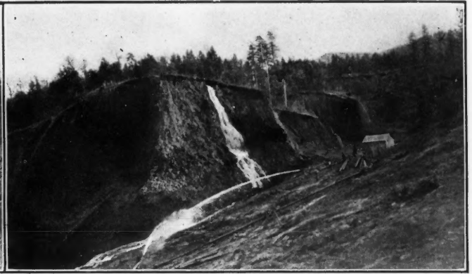
The Osgood is the only mine at Waldo having sufficient grade to dispense with elevators for disposing of tailings
