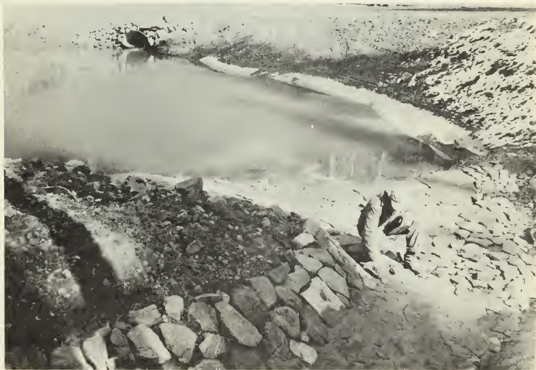
Pond of \frac{1}{4} acre-foot capacity in which to trap sediment
