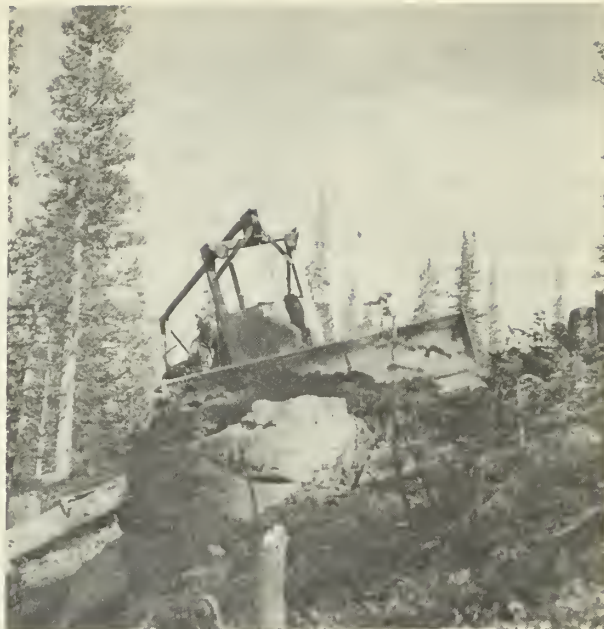
Constructing a logging road with a bulldozer
