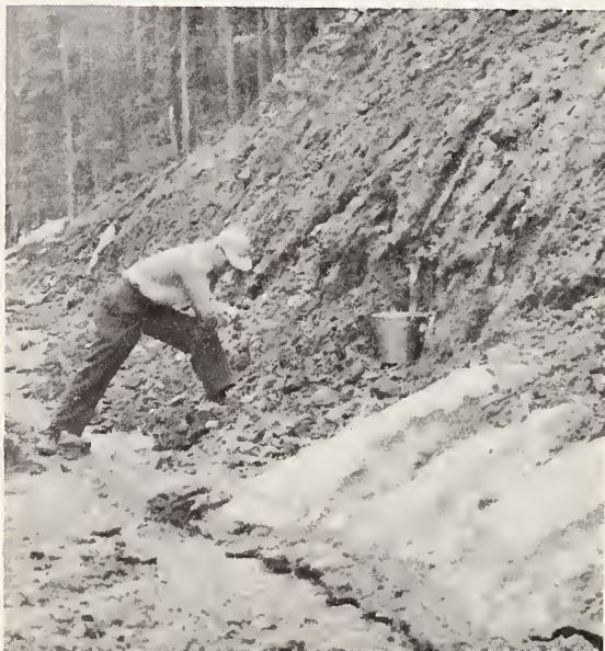
Flow of water along a deep clay layer in the soil exposed by a road cut
