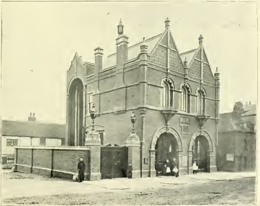
THE NEW FIRE STATION.
