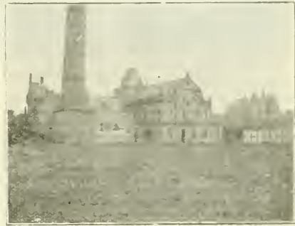
EDINBURGH: GENERAL VIEW OF THE POWDERHALL REFUSE DESTROYER BUILDINGS FROM THE NORTH.
