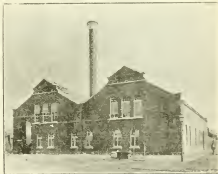
CORK ELECTRIC TRAMWAYS: POWER-HOUSE.
