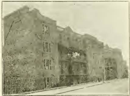
EDINBURGH: SOUTH FRONT OF TENEMENTS AT HIGH SCHOOL-YARDS.
