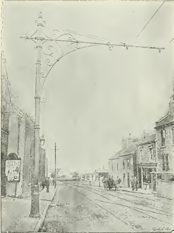
BRISTOL ELECTRIC TRAMWAY: SIDE POLE AND BRACKET.
