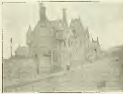
EDINBURGH: POWDERHALL REFUSE DESTROYER WORKS, EAST FRONT OF STABLING, ETC., TOWARDS BROUGHTON ROAD.
