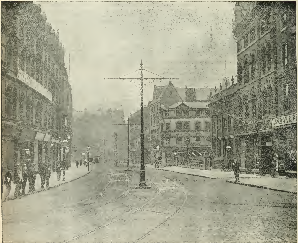
LEEDS CITY TRAMWAYS : CENTRE POLES IN BOAR-LANE. (Trolley wires not in position.)
