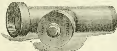
Fig. 2.—Joiner on Junction.
