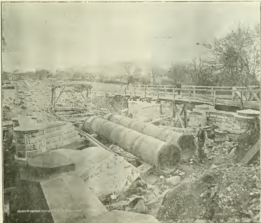
CAETHON SIPHON STREAM CROSSING, LOOKING EAST (February, 1907).
