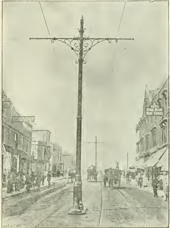
BRISTOL ELECTRIC TRAMWAY: CENTRE POLES AND BRACKETS.
