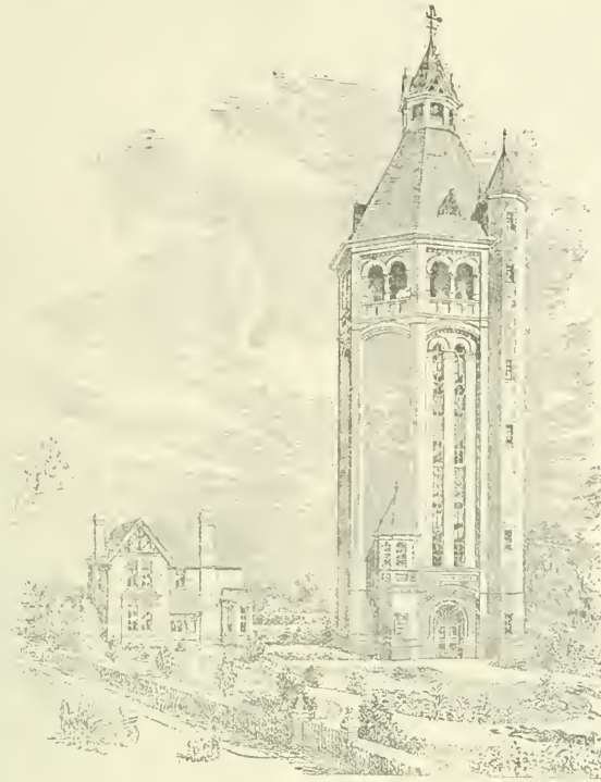
LEIGHTON BUZZARD WATER TOWER: GENERAL VIEW.
