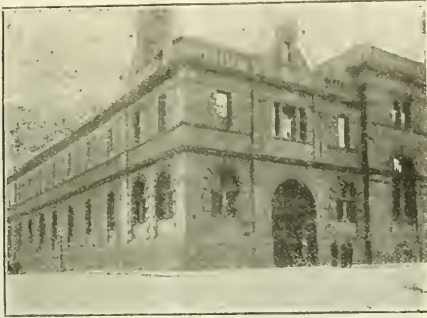
EDINBURGH: NORTH FRONT AND END OF BOILER-HOUSE AND COAL STORE AT THE CENTRAL ELECTRIC LIGHTING STATION.
