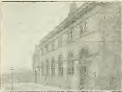
EDINBURGH: WEST FRONT OF CENTRAL ELECTRIC LIGHTING STATION (ENGINE ROOMS, &c.).
