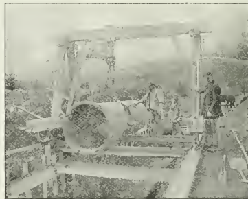
WYE SYPHON, PREPARING TO LOWER A PIPE (February, 1897).
