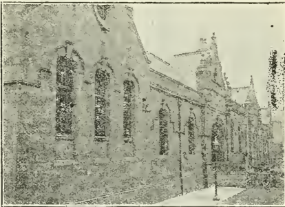
EDINBURGH: TOLL-CROSS CABLE-POWER STATION, SOUTH FRONT OF CAR SHEDS.
