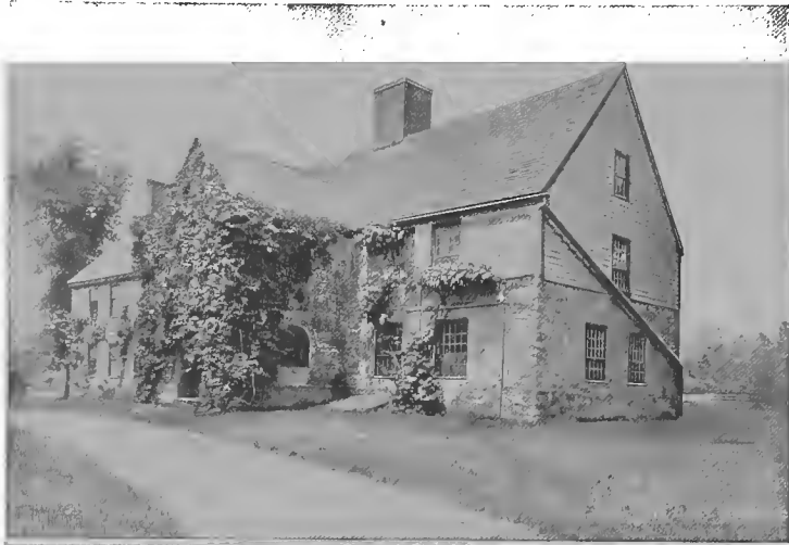
SPENCER-PIERCE HOUSE, NEWBURY (CIR. 1650)
