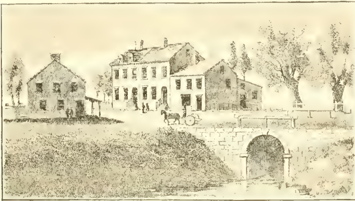
STONE BRIDGE WHERE BROADWAY NOW CROSSES CANAL STREET
