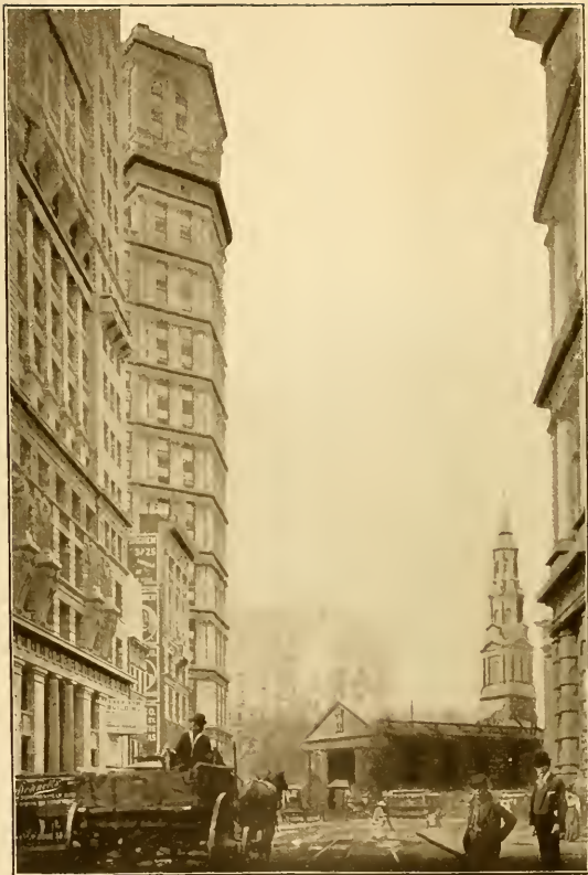
ST. PAUL'S CHURCH, FROM PARK ROW. NORD-ANSICHT DER ST. PAUL'S KIRCHE.
