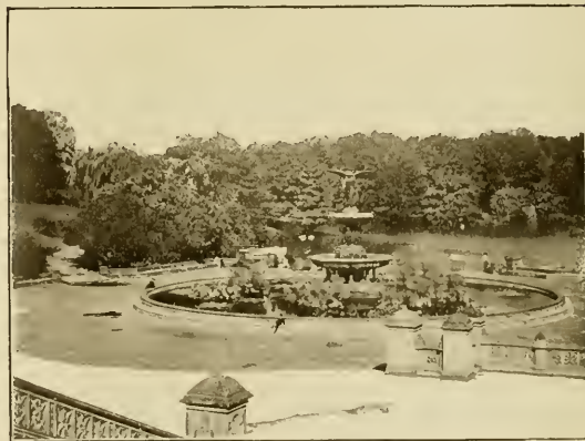
BETHESDA FOUNTAIN, CENTRAL PARK. BETHESDA SPRINGBRUNNEN IM CENTRAL PARK.
