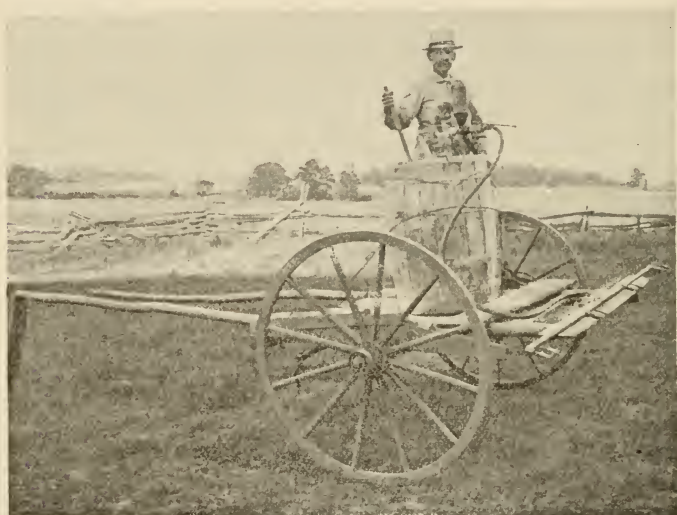
100.—An excellent home-made potato sprayer, treating four rows.
