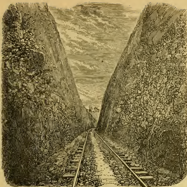
NO. III.—BLOOMER CUT, (63 feet deep, 800 feet long.)
