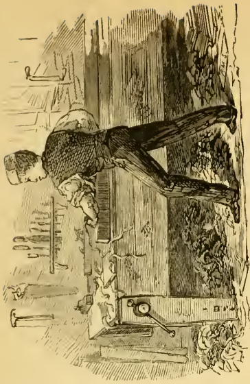
GETTING OUT FLOOR BOARDS BY HAND. Planer gets out ten thousand feet. Two hundred feet a day's work.
