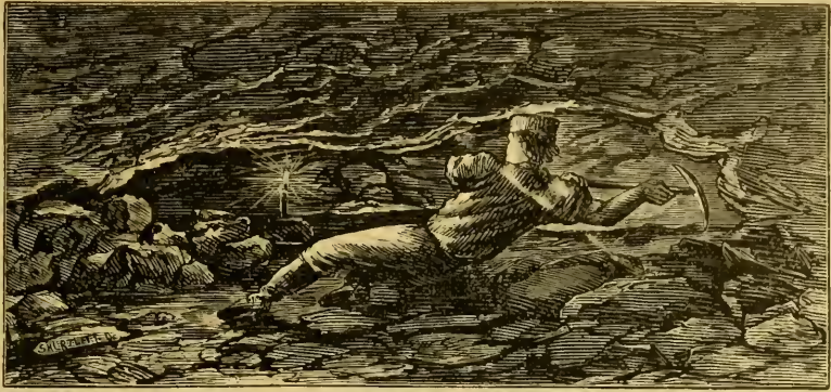
UNDERMINING COAL.—See page 141.
