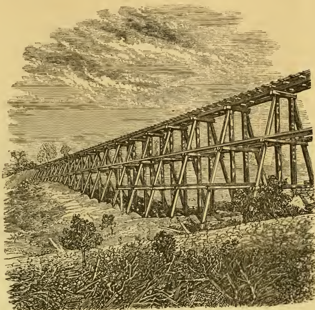
NO. I.—TRESTLE OPPOSITE AUBURN.
