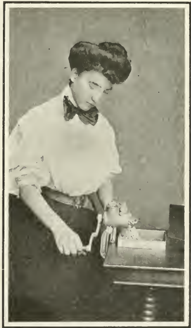
Fig. 263—Grinding the paper pulp
