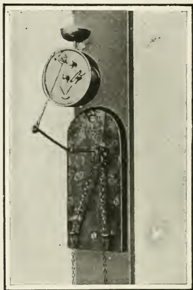
Fig. 288—Drafts closed, alarm set
