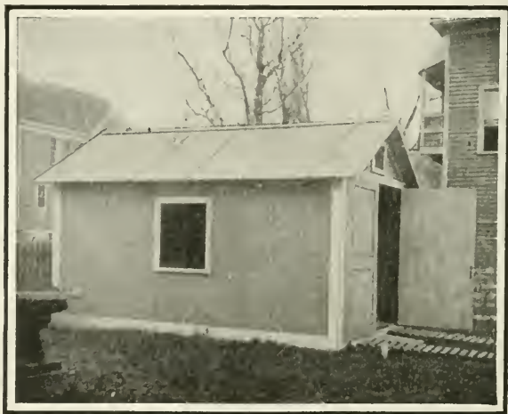
Fig. 309—A side view of the portable automobile house
