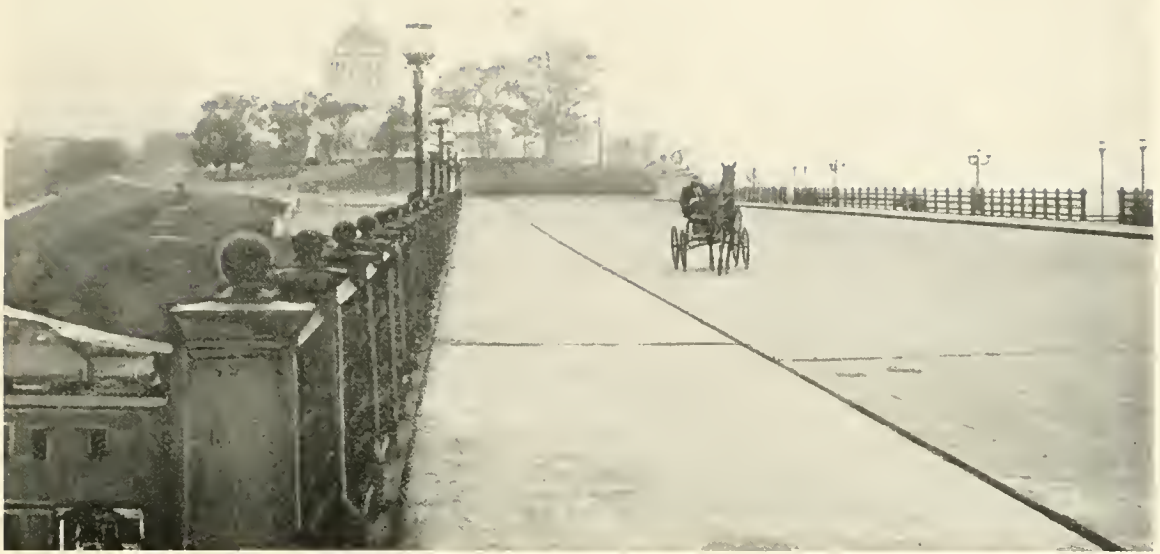
RIVERSIDE DRIVE VIADUCT.
