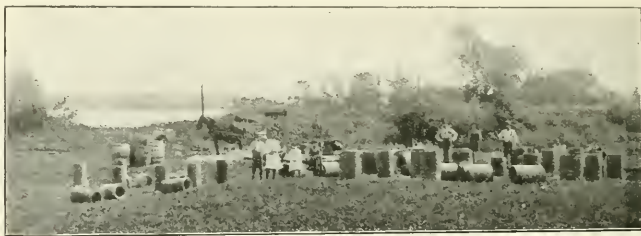
MAKING CONCRETE CULVERT PIPE.
