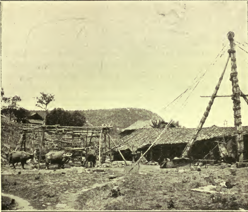
BORING FOR SALT AT TZELIUTSING.
