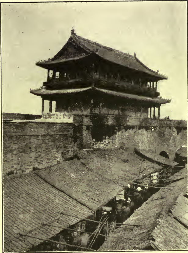
THE EAST GATE, CHENGTU, WITHOUT THE WALL.
