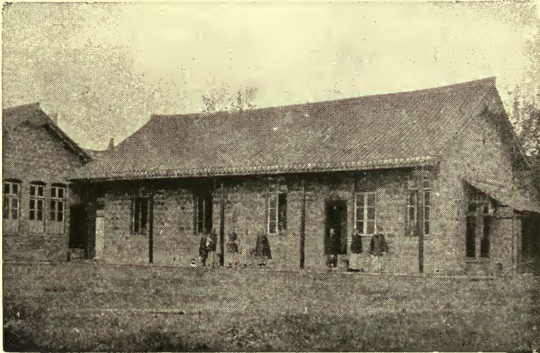
OUR FIRST HOSPITAL IN WEST CHINA.
