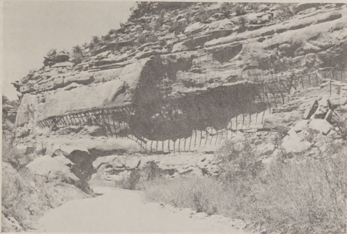
The 6-mile-long hanging flume near the confluence of the San Miguel River once carried water for gold mining.
