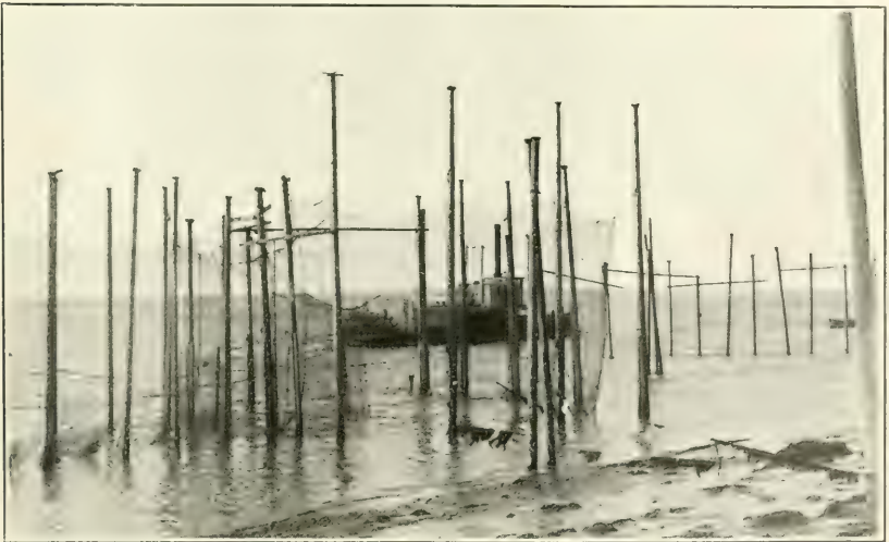
A TYPICAL SALMON TRAP NEAR GRAVEYARD POINT, KIRCHAK BAY, SHOWING THE NORTHERN AND INSHORE POT, AS SEEN FROM THE BEACH AT LOW TIDE, THE TUNNEL BEING DOWN
