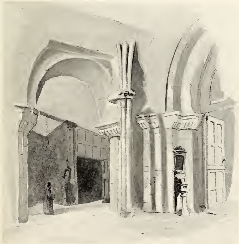
WEST END OF SOUTH AMBULATORY (see pp. 25, 142, 339, 348)
