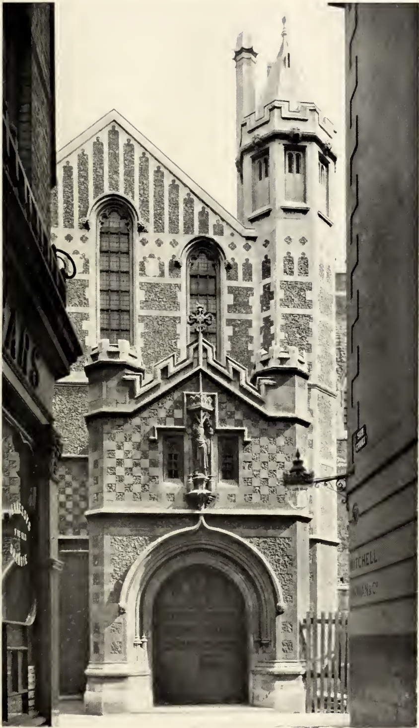
NORTH TRANSEPT, PORCH, AND TURRET (see pp. 51, 106, 118)
