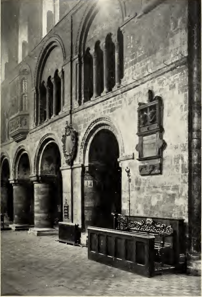
GROUND ARCADE, SOUTH SIDE OF QUIRE (see pp. 8, 16)
