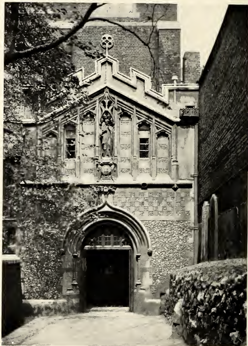
WEST PORCH (see pp. 106, 109)
