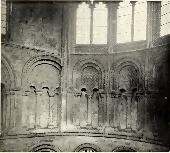
TRIFORIUM: JUNCTION OF NEW WITH OLD WORK (see pp. 12, 32)
