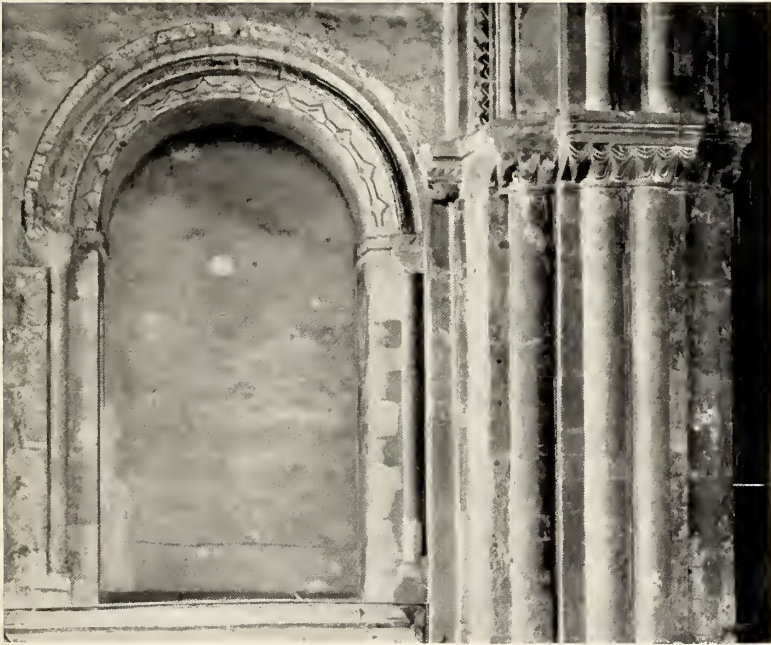
TRIFORIUM: SOUTH TRANSEPT AND SOUTH-WEST PIER OF CROSSING (see pp. 8, 44, 54, 55, 56)
