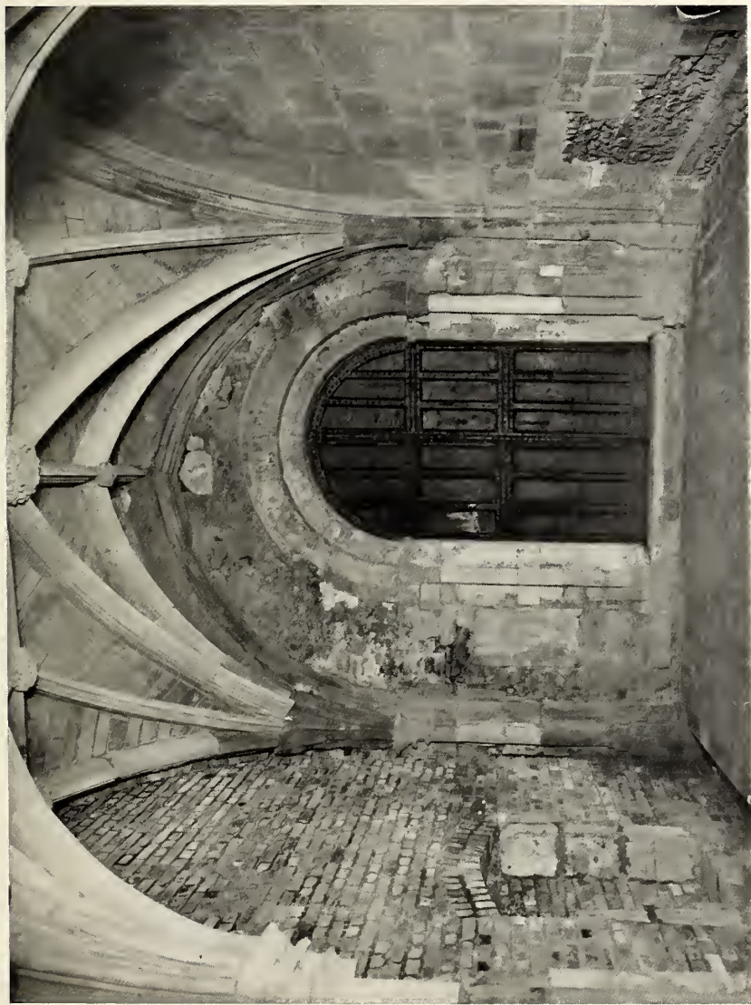
EAST WALK OF CLOISTER, LOOKING NORTH (see pp. 9, 14, 65, 132, 141)
