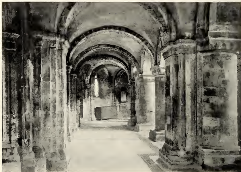
NORTH AMBULATORY, LOOKING EAST (see pp. 7, 24, 29)
