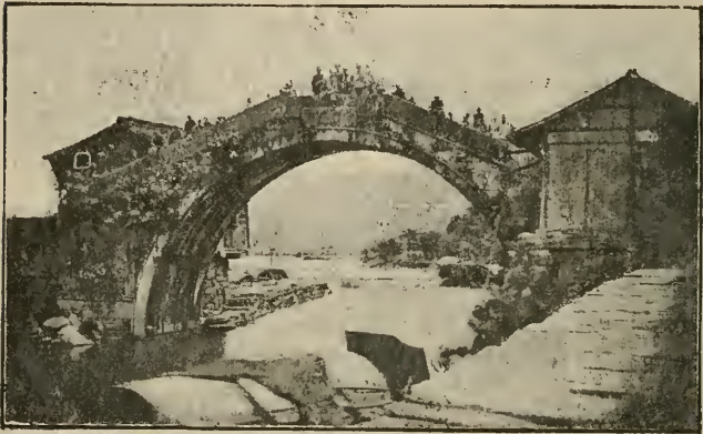
BRIDGE AT NING-KONG-GYIAO.
