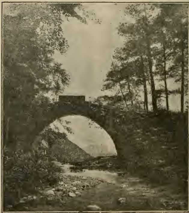
BRIDGE NEAR WUN-CHAU.
