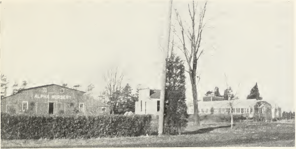
Office, Greenhouse and Packing Sheds.
