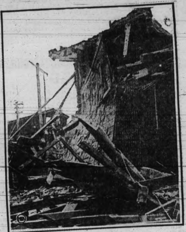
NEW QUAKE WRECKED THIS. —This picture gives an idea of the violence of Japan's most recent earthquake, that of Jan. 15. It shows the ruins of Wadakra Gate, one of the entrances to the Imperial Palace in Tokyo. The gate withstood the September tremor.
