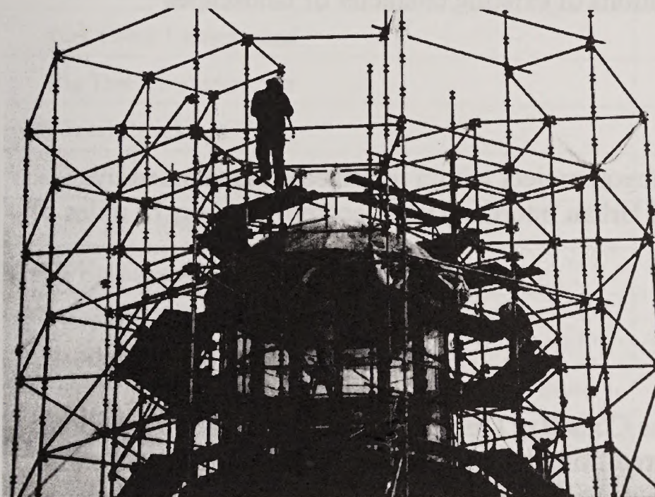
Repairing the roof on the Cape Blanco Lighthouse
