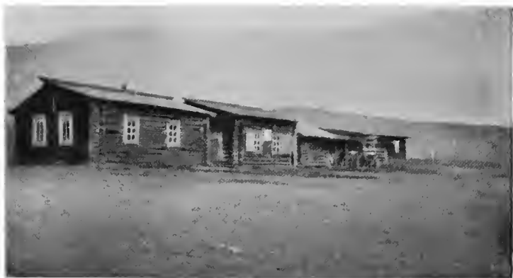
HOUSE WHERE WE BOARDED ON OLKHON ISLAND. Page 72 The building with the white sign is the Russian store
