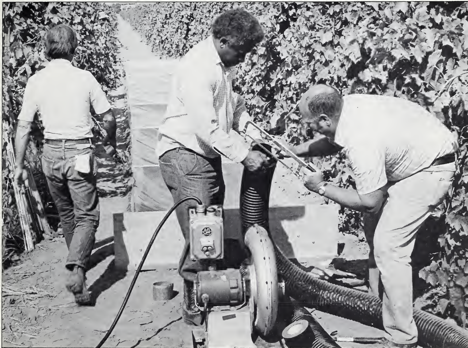
Above: Food technologist Rogernald Jackson holds while Huxsoll trims plastic tubing for a snug fit onto an electric blower used to circulate air between the polyethylene sheets of his field-constructed solar tunnel (0980X1168-4).
