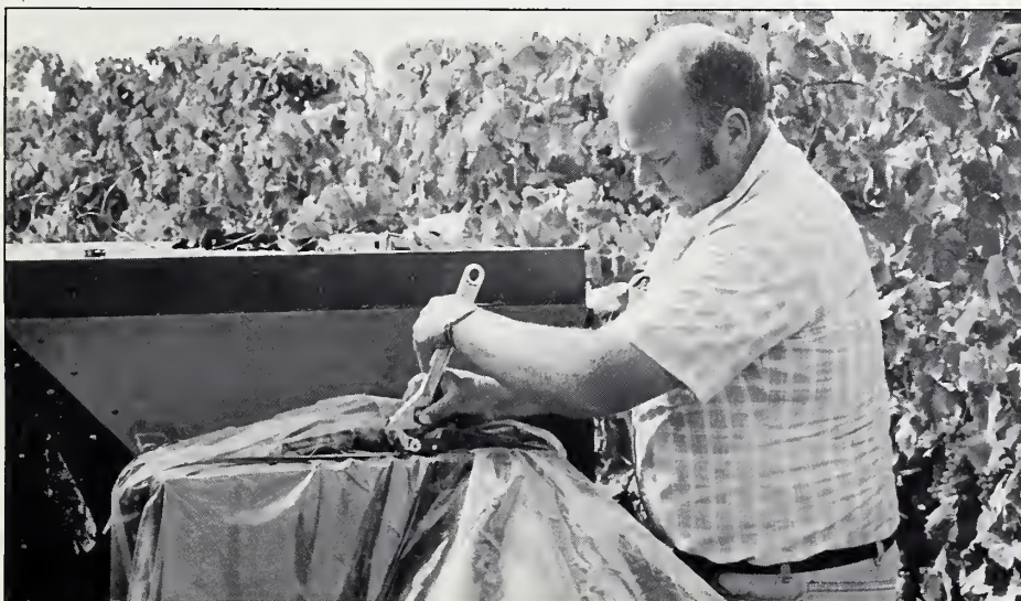
Above: Food technologist Rogernald Jackson holds while Huxsoll trims plastic tubing for a snug fit onto an electric blower used to circulate air between the polyethylene sheets of his field-constructed solar tunnel (0980X1168-4).
