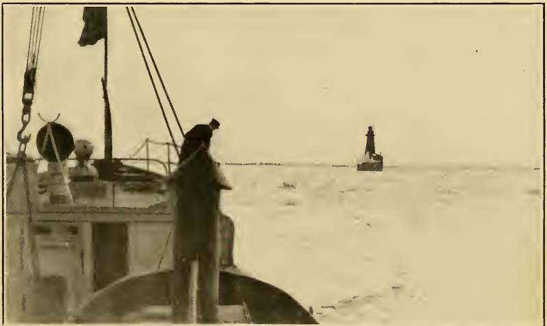
FIG. 10.—Lake Superior on May 7, 1923, still jammed with ice. Stannard Rock Light, on the right, is one of the most interesting lighthouses on the Lakes, inasmuch as it is built on a submerged rock, 28 miles from land, and is surrounded by depths of 400 or 500 feet
