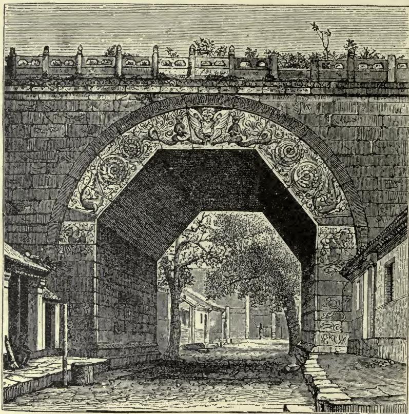
ARCHWAY IN THE GREAT WALL.
