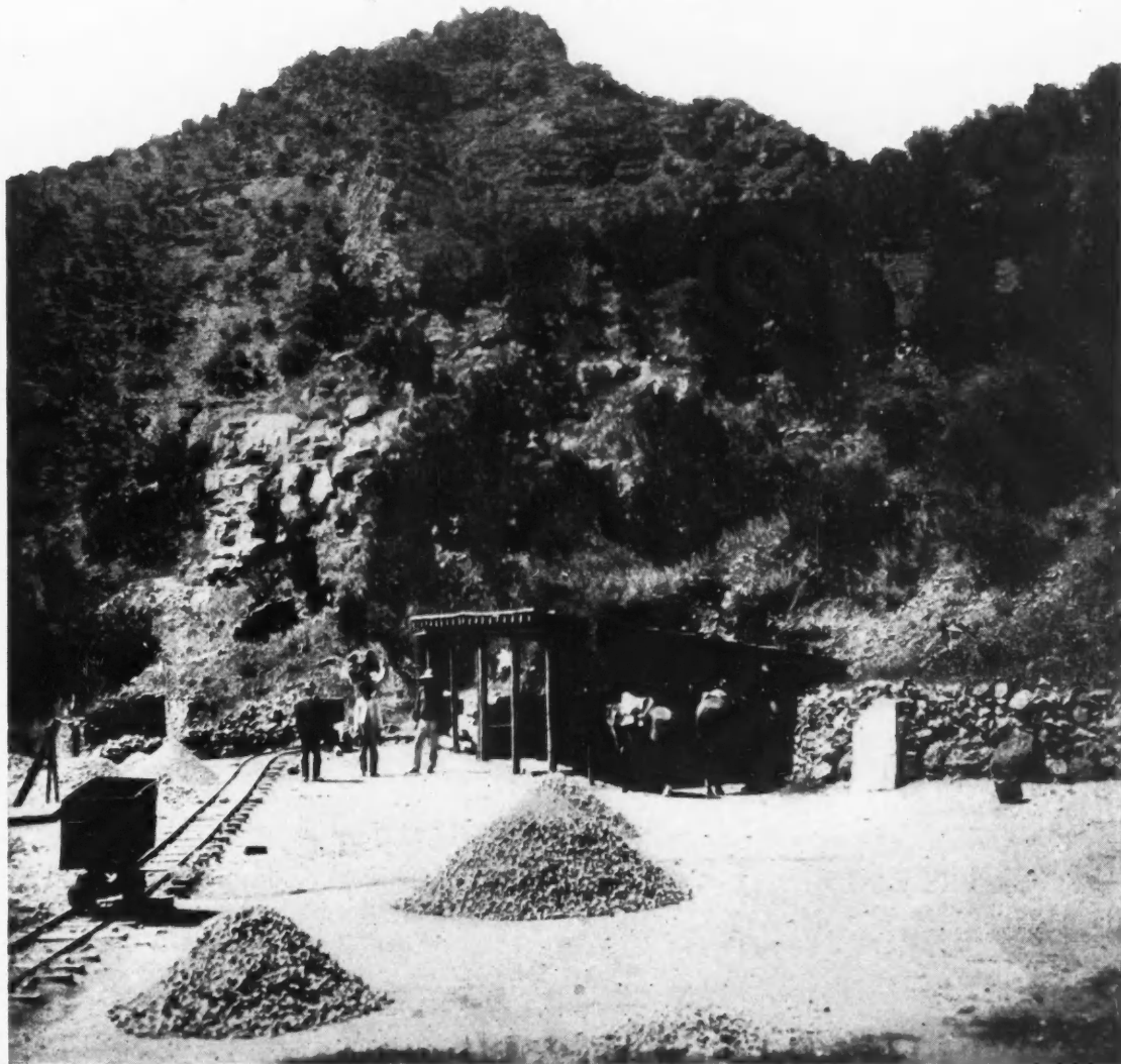
Entrance to adit, San Jose mine, Guanacevi camp, Durango, Mexico. San Marcos outcrop in background
