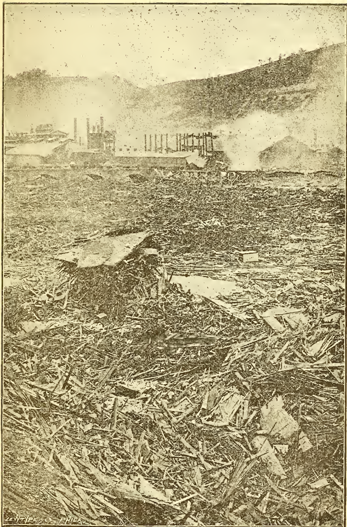
THE DÉBRIS ABOVE THE PENNSYLVANIA RAILROAD BRIDGE.
