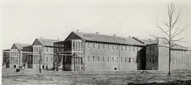
THE NEW DETACHMENT BARRACKS
