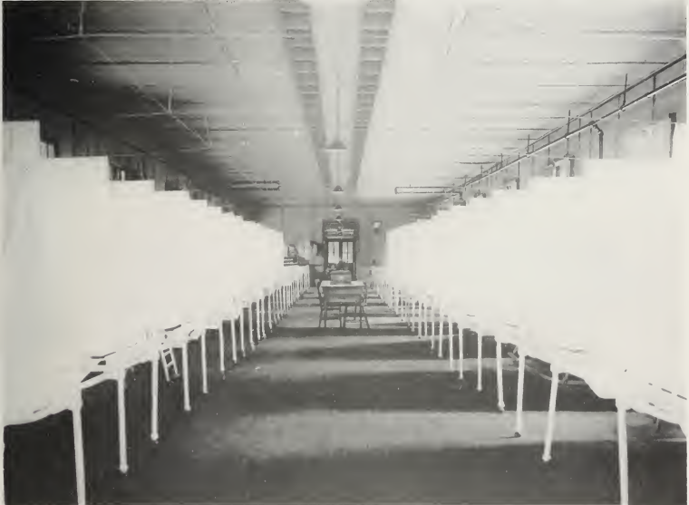
INTERIOR OF A WARD
