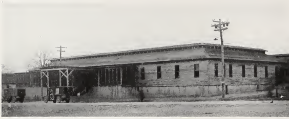
THE RECEIVING WARD BUILDING
