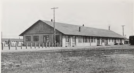
THE CAMP RAILROAD STATION
