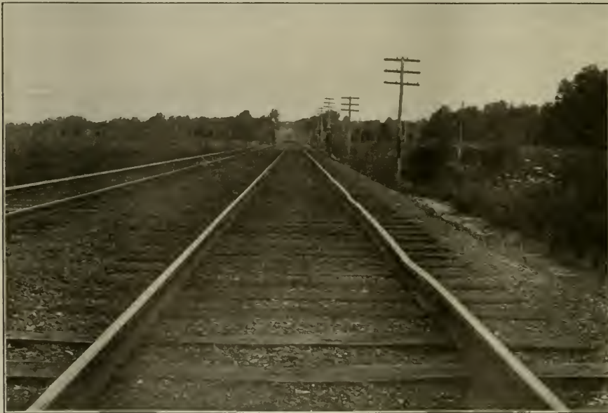
EFFECT OF A HEAVY ILL-BALANCED LOCOMOTIVE ON RAILROAD TRACK.
