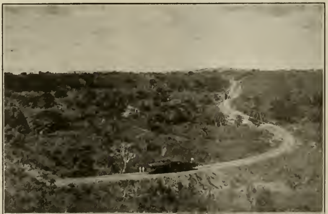
CHIRIQUI NATIONAL RAILWAY, PANAMA CANAL ZONE, RIO DAVID VALLEY.
