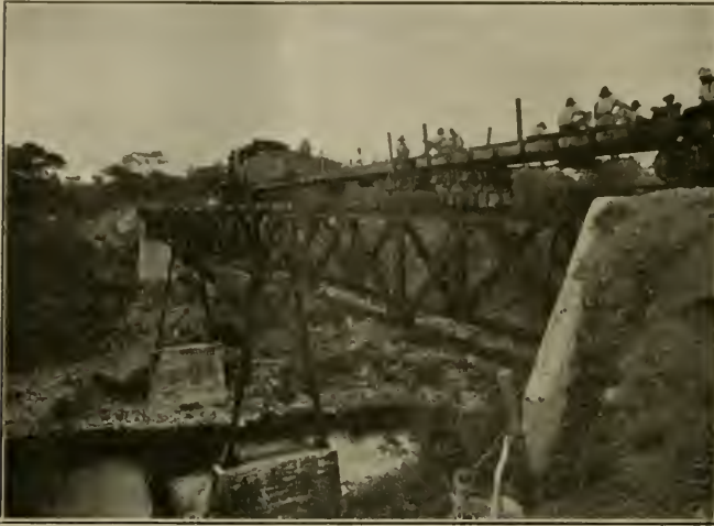
RIO MAJAGUA BRIDGE—CHIRIQUI NATIONAL RAILROAD.
