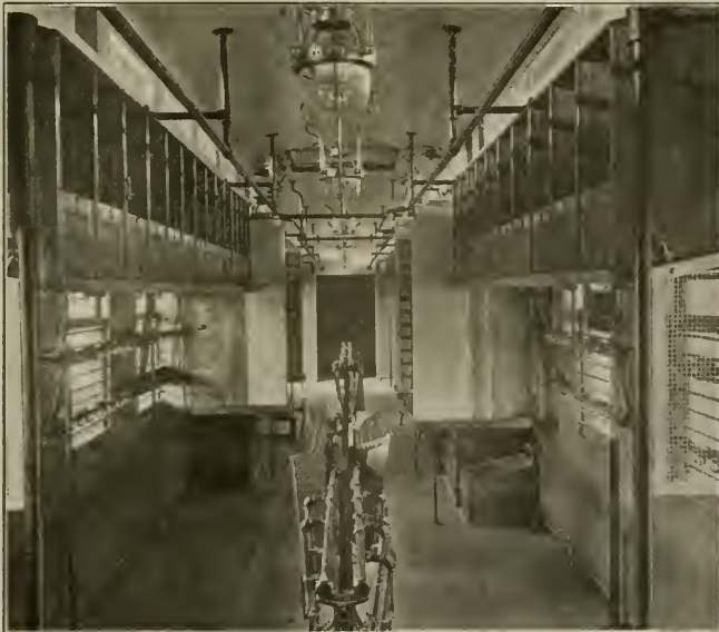
INTERIOR OF B. & M. STEEL POSTAL CAR
