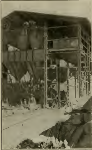
BRAZILIAN COAL GRINDING PLANT IN COURSE OF ERECTION.
