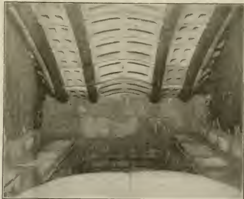
SECURITY BRICK ARCH FORMING FURNACE FOR PULVERIZED FUEL.
