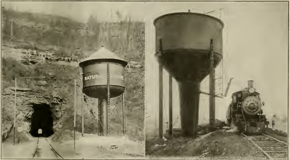
CONICAL TANK BOTTOM, L. & E. RY.
