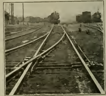
SWITCH SET FOR SIDE TRACK SERVICE of anthracite buckwheat and bituminous coals to make the mixture.
