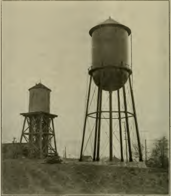
ORDINARY WOODEN TANK AND HEMISPHERICAL BOTTOM STEEL TANK WITH CAPACITY OF 200,000 GALLS. 51 FT. 6 INS. HIGH.
