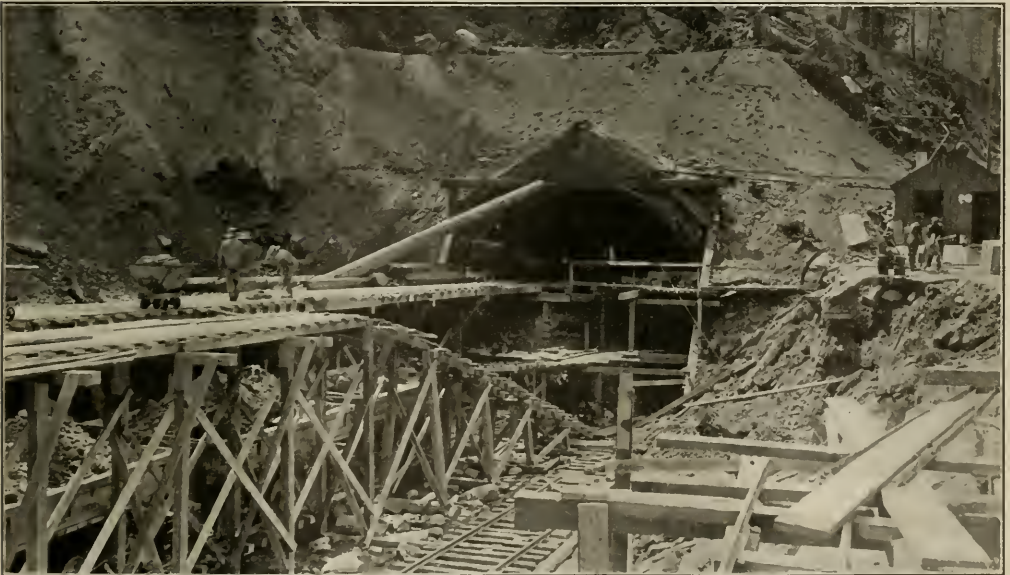
PORTAL OF THE CONNAUGHT TUNNEL DURING CONSTRUCTION. CANADIAN PACIFIC RAILWAY.
