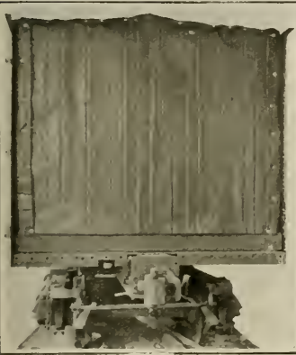
END VIEW P. R. R. REFRIGERATOR CAR—SIDE SHEATHING PLACED.
