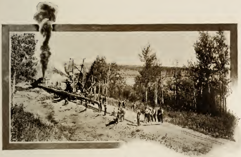
RAILWAY BUILDING IN SASKATCHEWAN
