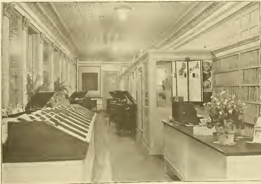
A COMPLETE CURRY INSTALLATION
