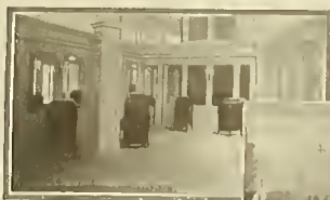
Machines Display Rooms
