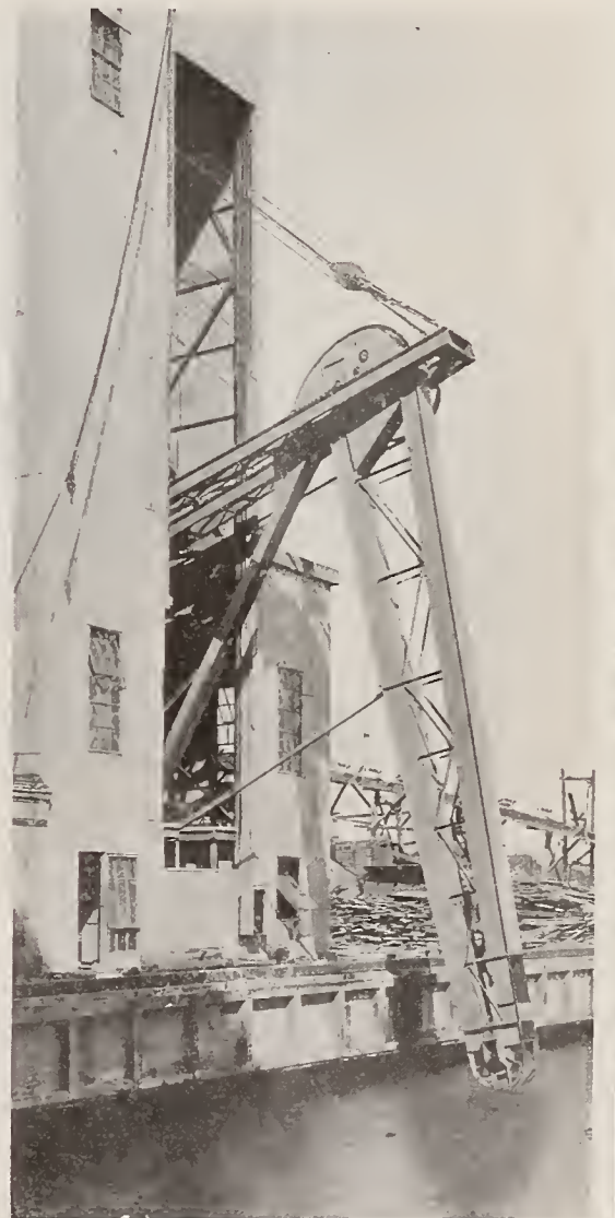
MARINE LEG NORTHERN CENTRAL ELEVATOR BALTIMORE, MD.
