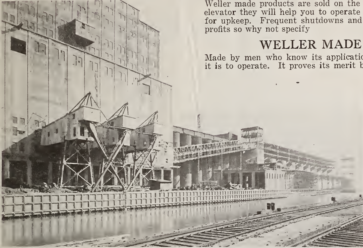
NORTHERN CENTRAL ELEVATOR, BALTIMORE, MD.
