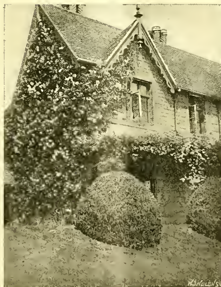
FIG. 46.—THE GARDENER'S COTTAGE AT LINTON PARK, NEAR MAIDSTONE.
